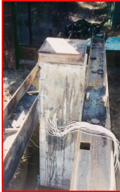
b) End of driving of prestressed pile showing driving cushion compressed
