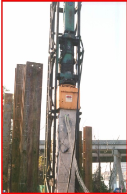
a) Driving of prestressed pile
