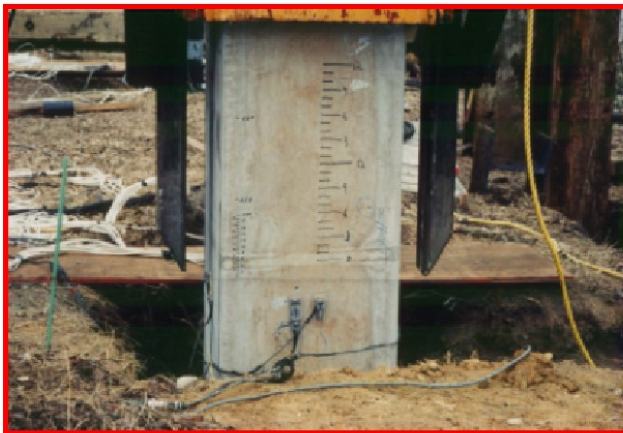
c) Restrike of prestressed pile
