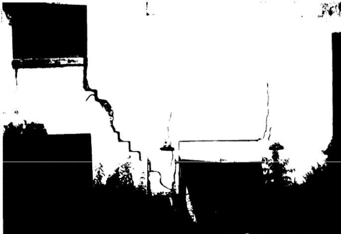
b. Diagonal and vertical cracks
