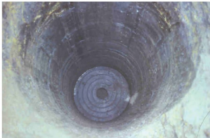
Figure 4-1 Dry Hole in Stable Soil
