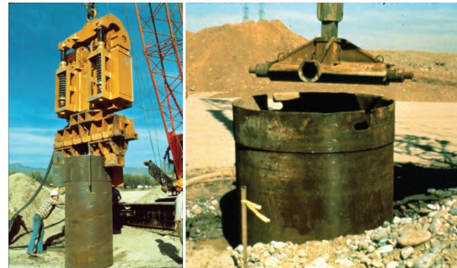
Figure 4-10 Use of a Vibro-Hammer (Left) and Twister Bar (Right) to Advance Casing
