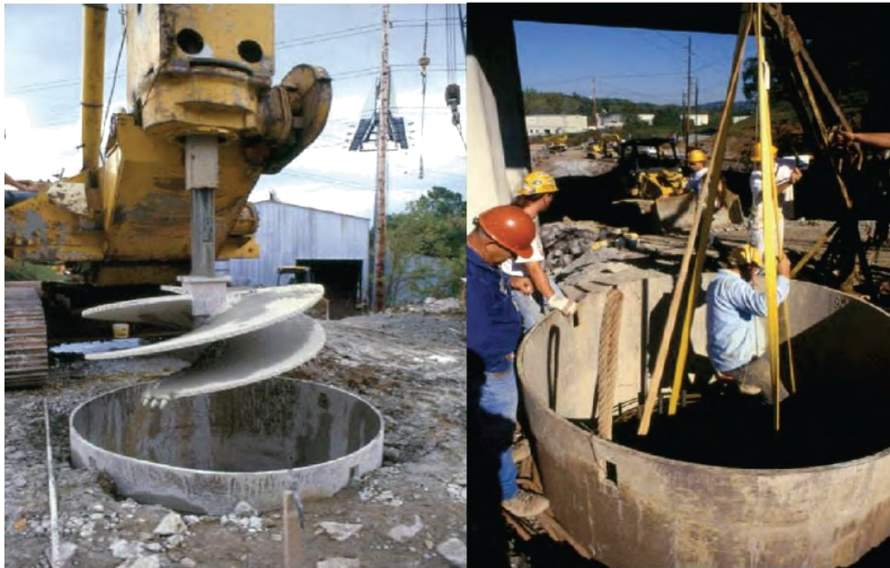
Figure 4-6 Drilling into Rock through a Cased Hole
