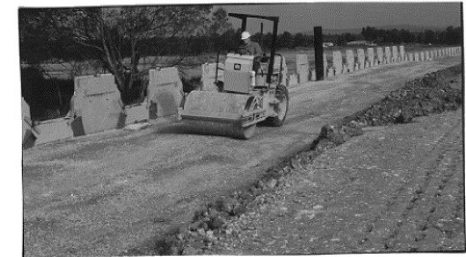
Figure 13. Compaction of backfill.
