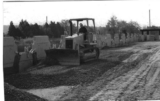
Figure 13. Compaction of backfill.
