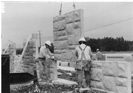
Figure 11. Erection of precast panels.
