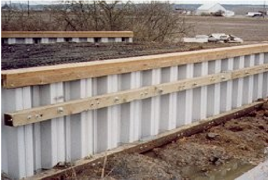
Anchored sheet pile walls
