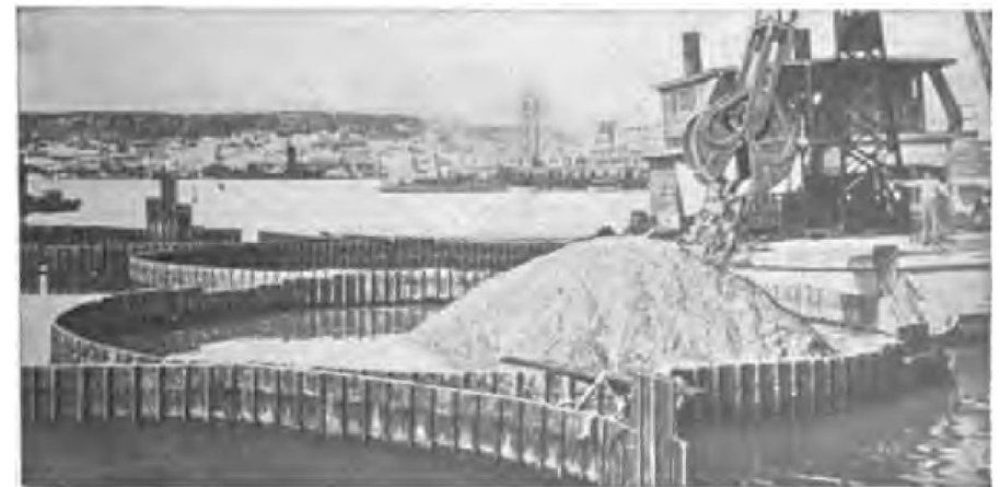
FIG. 71g.—Filling Clay into Cylinder A. Part of B in Foreground.
