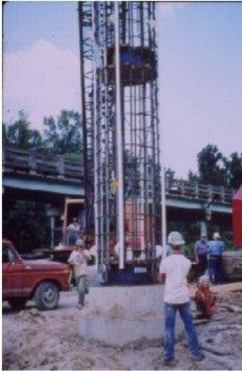
Figure 38, Osterberg Load Cells
