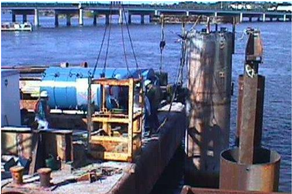
Figure 37, Lateral Static Load Test
