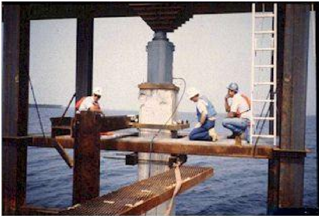
Figure 35, Static Load Test
