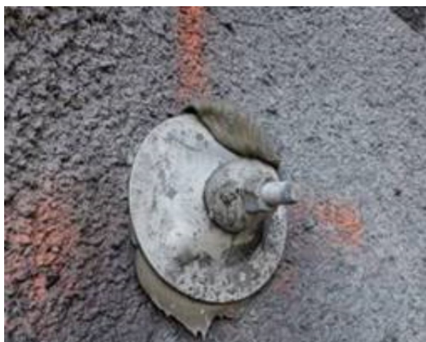
Figure 4.13 Bolt in cutting prior to tightening of the plate. This is done after the grout has cured. Photo Terje Kirkeby
