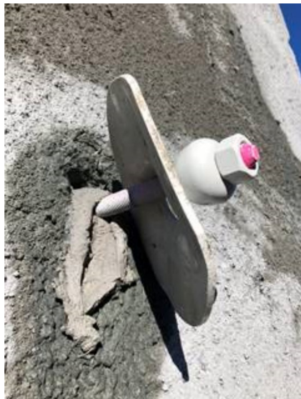
Figure 4.13 Bolt in cutting prior to tightening of the plate. This is done after the grout has cured. Photo Terje Kirkeby
