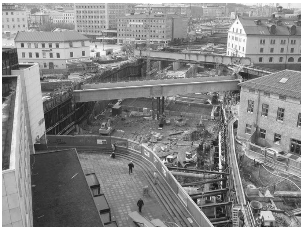
Figure 4.2. Overview of the excavation, March 2004
