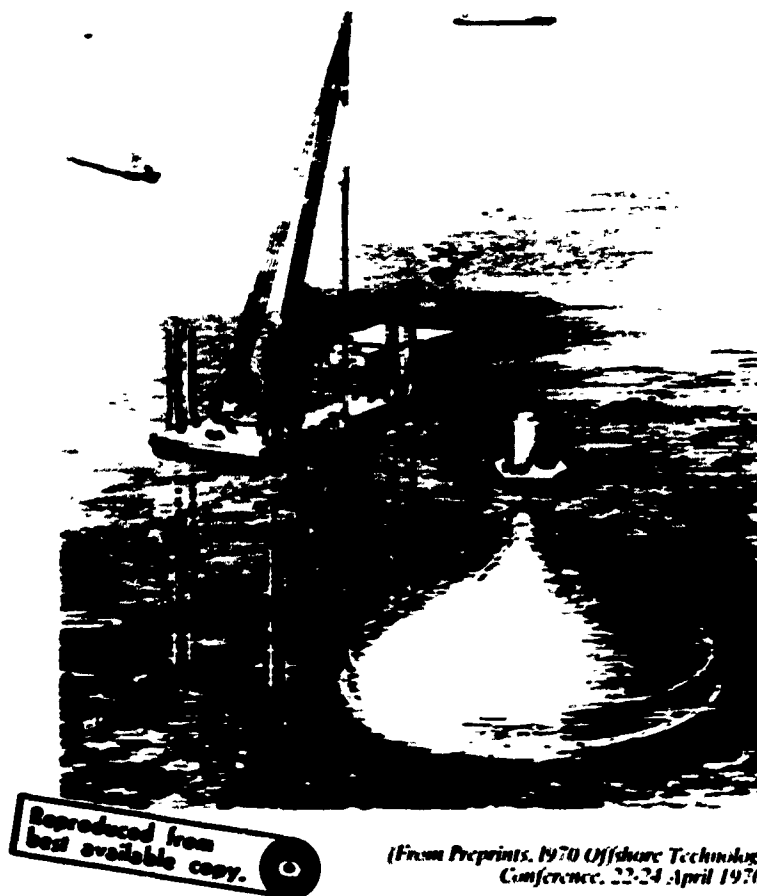
Fig. 64. Placing piles for the Khazzan Dubai 1 undersea storage tank (from reference 158)
