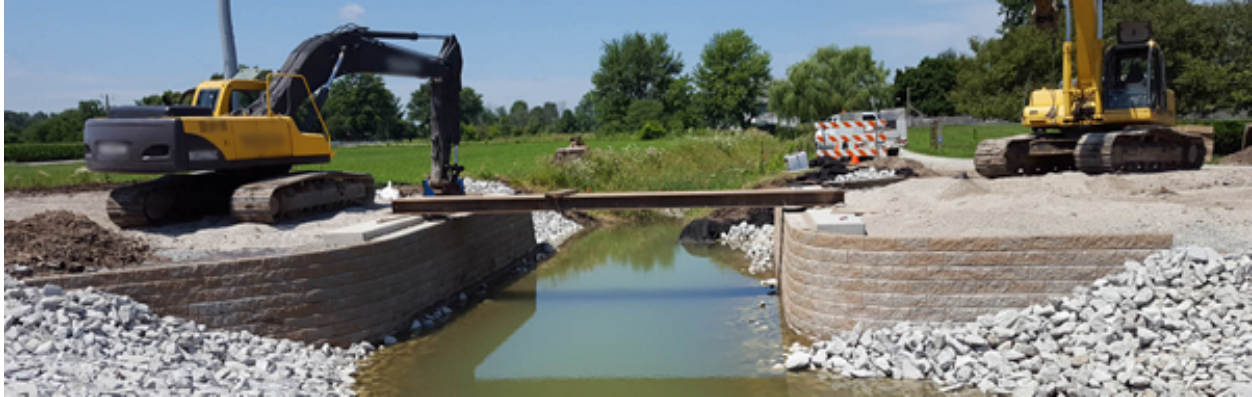
Figure 17. GRS abutments with rounded corners in Hamilton County, Indiana. Source: Hamilton County Highway Department.
