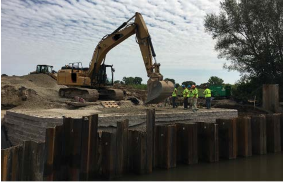
Figure 10. Cofferdam for a project in Dodge County, Wisconsin.
