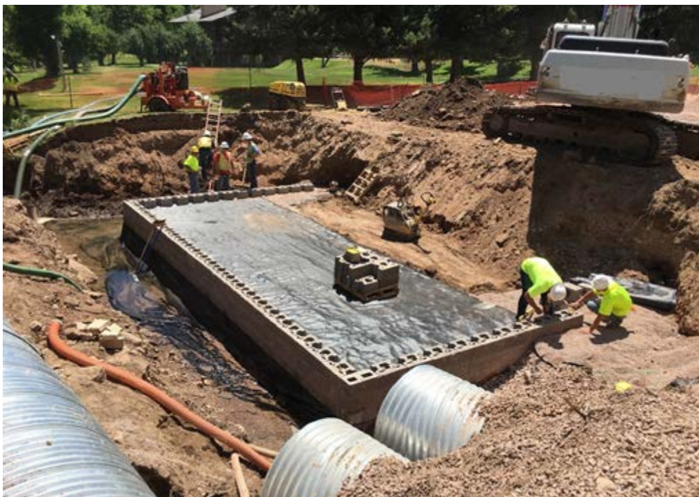
Figure 11. Dewatering area of excavation using culverts and pumps - Sand Creek Bridges Project in Crook County, Wyoming.
