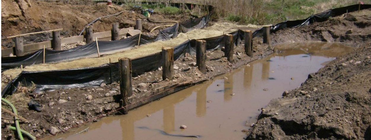
Figure 6. Timber piles from previous structure repurposed to provide temporary support for cast-in-place superstructure at State Highway 40 over Hay Creek Bridge. Source: Wisconsin Department of Transportation.
