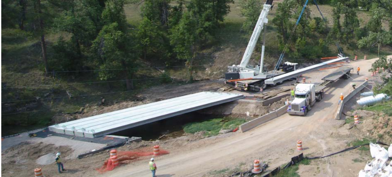
Figure 5. Placement of concrete girders on abutments at one of the Sand Creek Road Bridges in Crook County, Wyoming.
