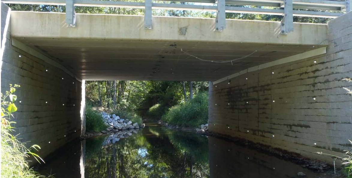
Figure 16. Surveying points installed on GRS wall facing.
