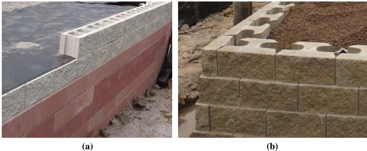
Figure 9. GRS abutment with split-face CMU block (a) and SRW block (b) facing.
