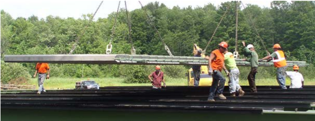
(a) Precast concrete panel lowered on top of steel girders
