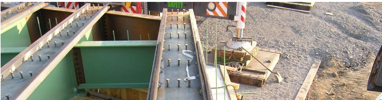
(b) Steel girder and precast concrete panel interface
