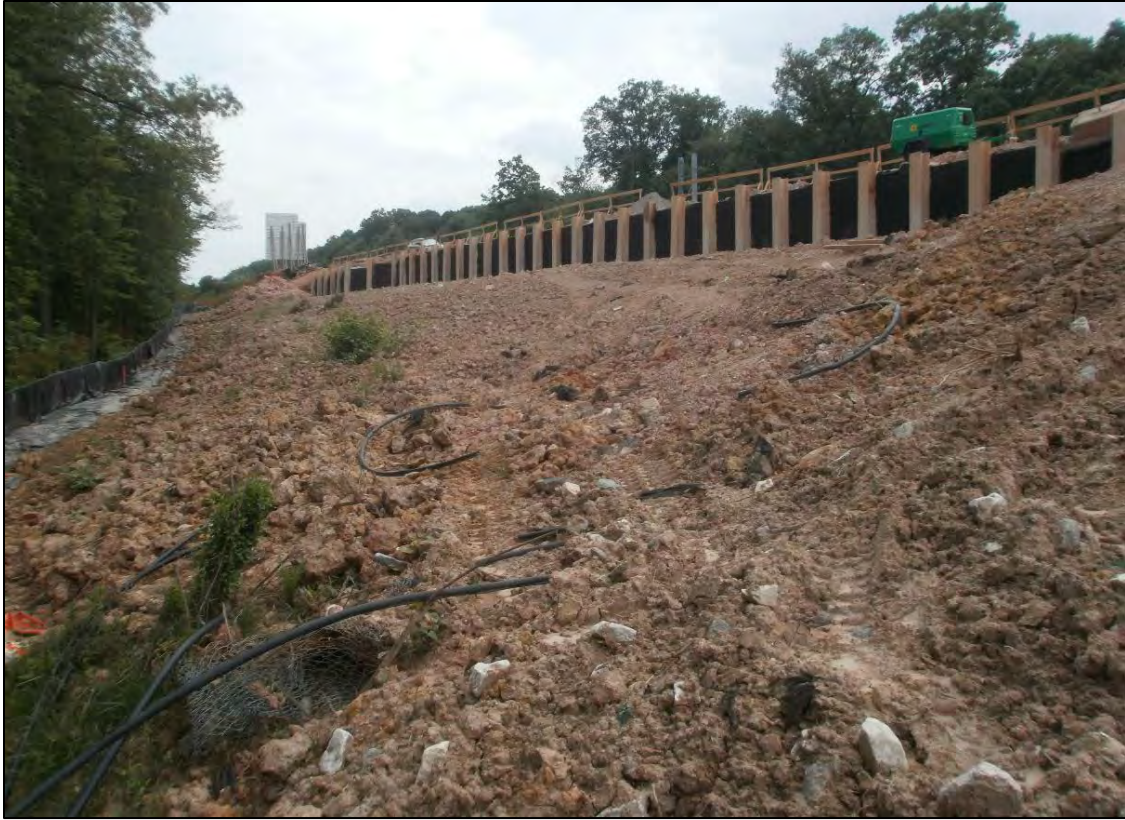
Figure 2-5: Slope stabilization with pile and lagging wall. (Soldier piles are embedded in drilled shafts extending below the slope failure surface)
