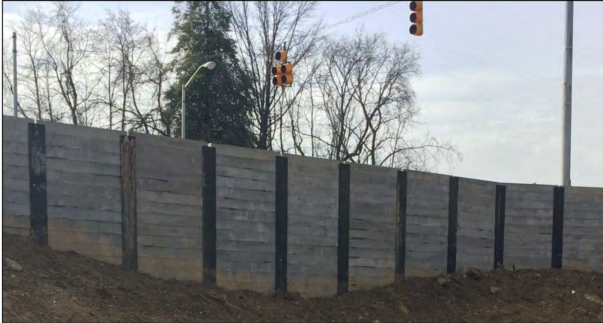
Figure 2-3: Permanent retaining walls: non-gravity cantilever wall.
