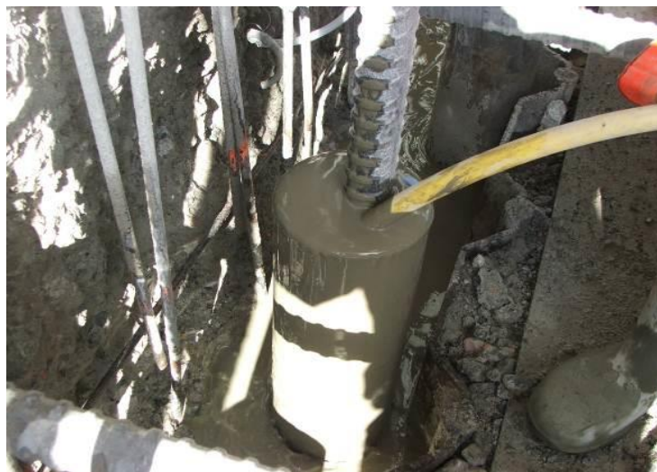
Figure 69. Photo. Grouting of micropiles
