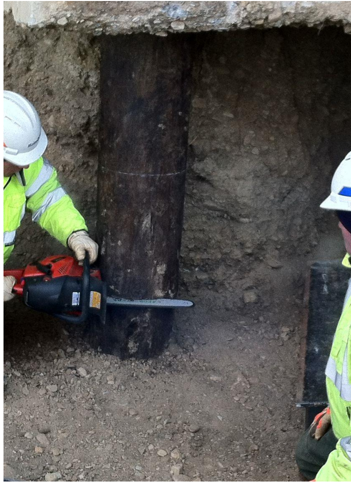
Figure 45. Photo. Excavation and removal of portion of timber piling at Haynesville Bridge
