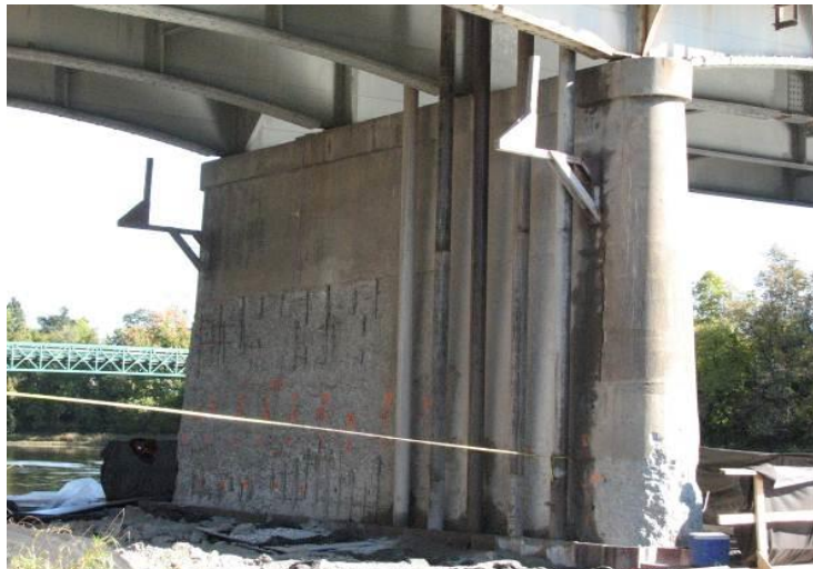
Figure 68. Photo. Micropile installation through bridge deck with casing down pier face
