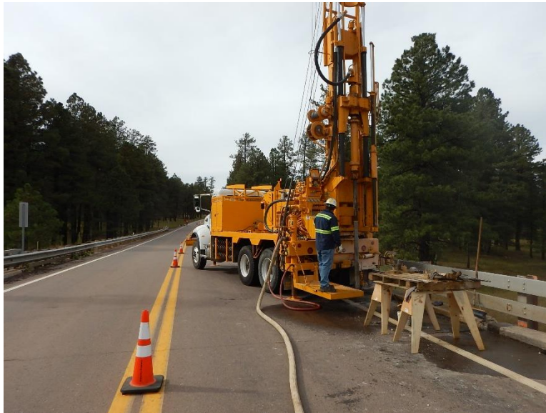
Figure 38. Photo. Coring through pier from bridge deck
