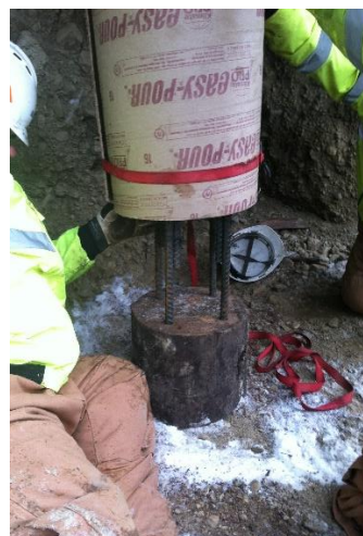
B. Repairing of a test pile with concrete
