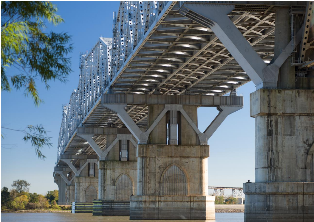
Figure 14. Photo. Huey P. Long Bridge with widened superstructure on reused foundation
