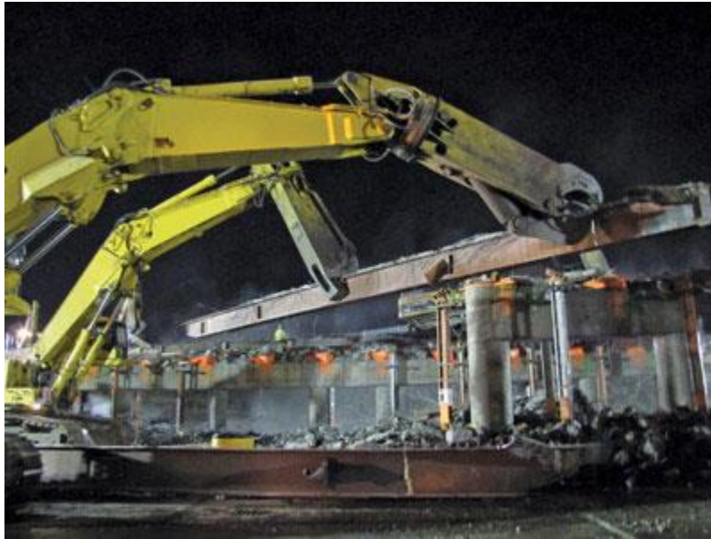
Figure 7. Photo. Demolition stage for removing the existing girders
