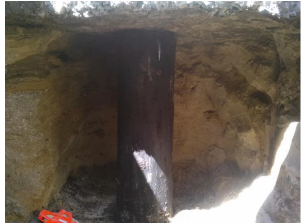
B. Timber pile at test pit 2
