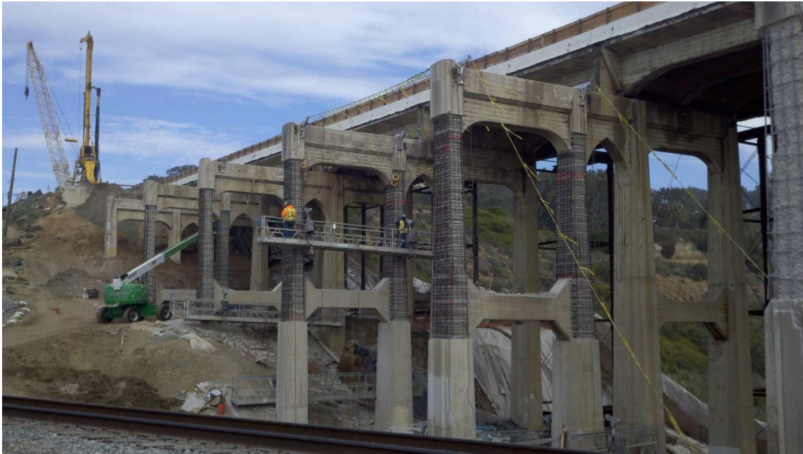
Figure 11. Photo. Installed column ties to increase the confinement of piers' columns
