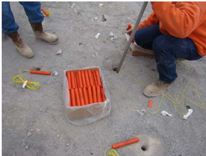
Figure 2-27. Primers with Caps Inserted Ready to Be Loaded Into Blastholes.
