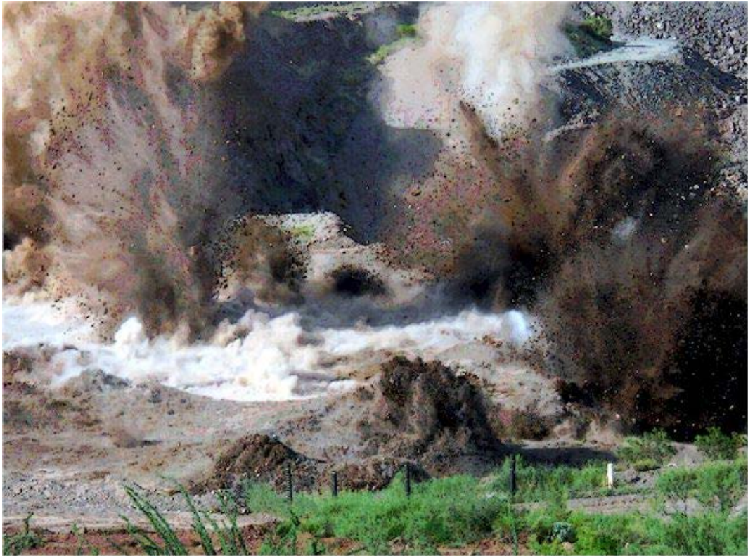
Figure 5-2. Flyrock Produced by a Blast with Excessive Burden and Over Confinement.
