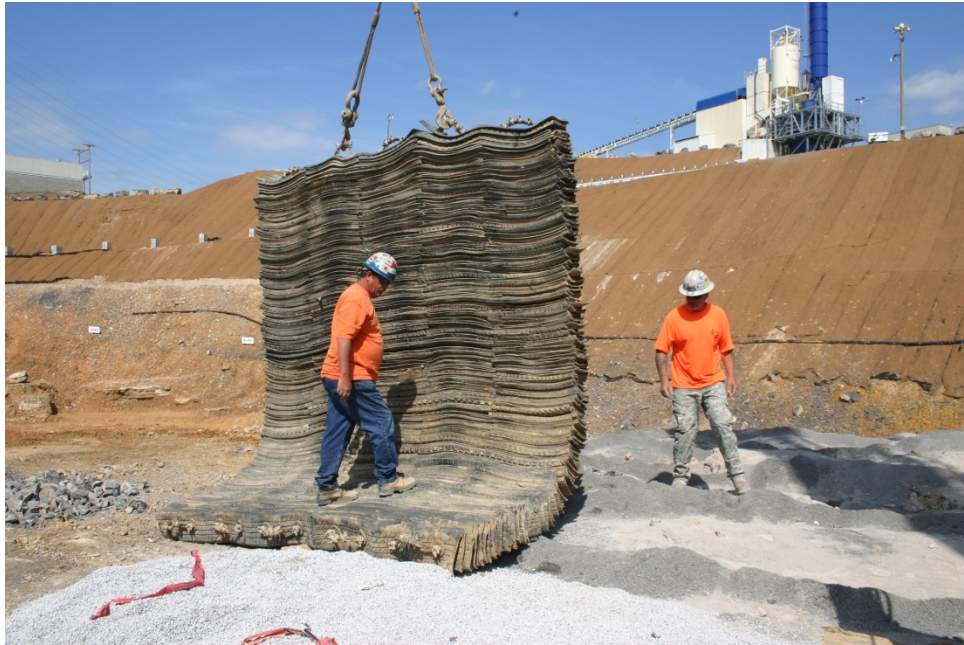
Figure 1-7. Rubber Blasting Mats Being Lowered Onto Shot at Kentucky Lock.
