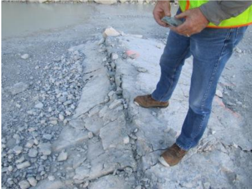
Figure 3-8. Heave in Quarry Floor Due to Unloading of the Rock by Blasting and Excavation.
