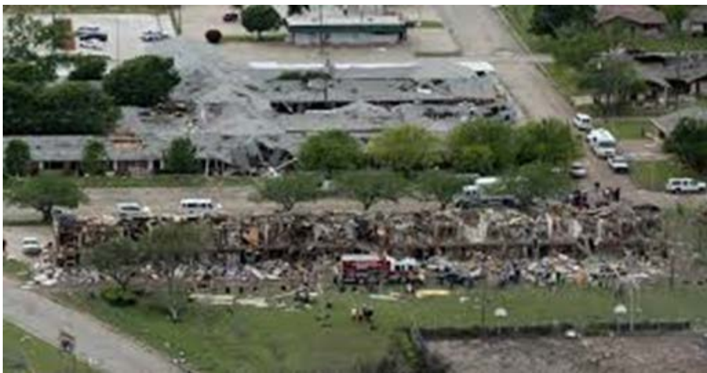
Figure 8-1. Airblast Damage at West, Texas Explosion.
