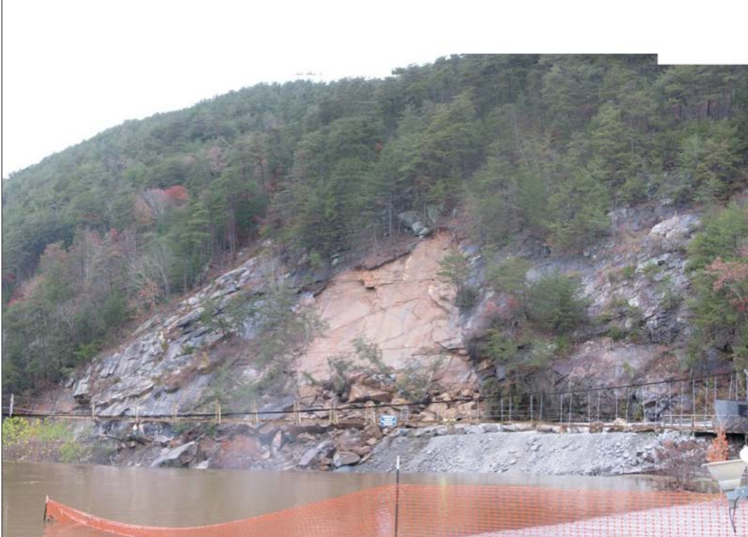
Figure 6-17. Rock Slide along US64 in the Ocoee River Gorge across from Parksville Dam, Immediately after the Slide.
