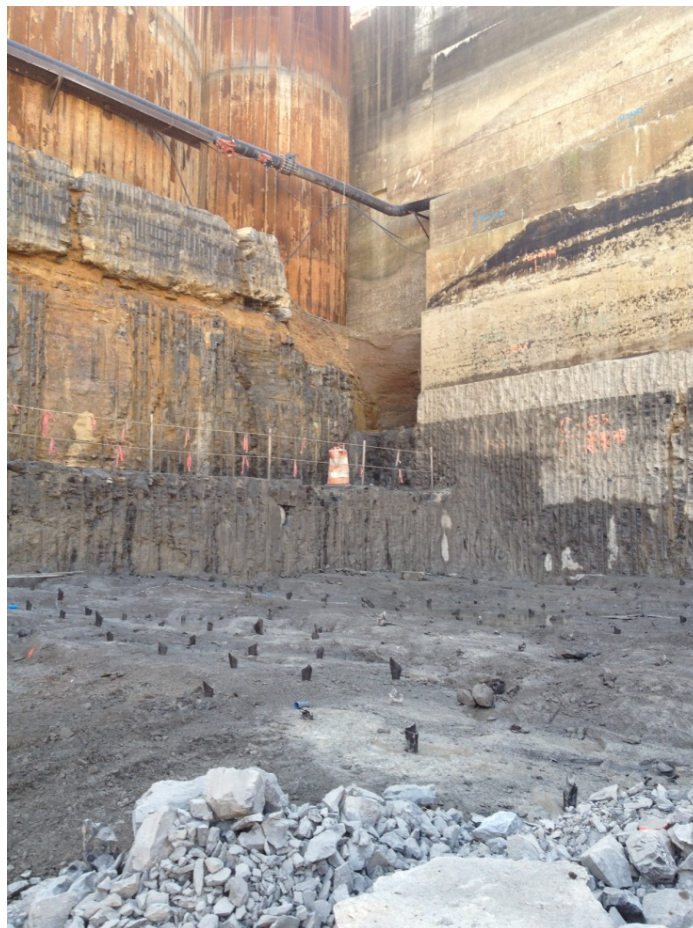
Figure 10-2. Photograph of Drilled Shot Pattern Also Showing Line Drilled Walls.
