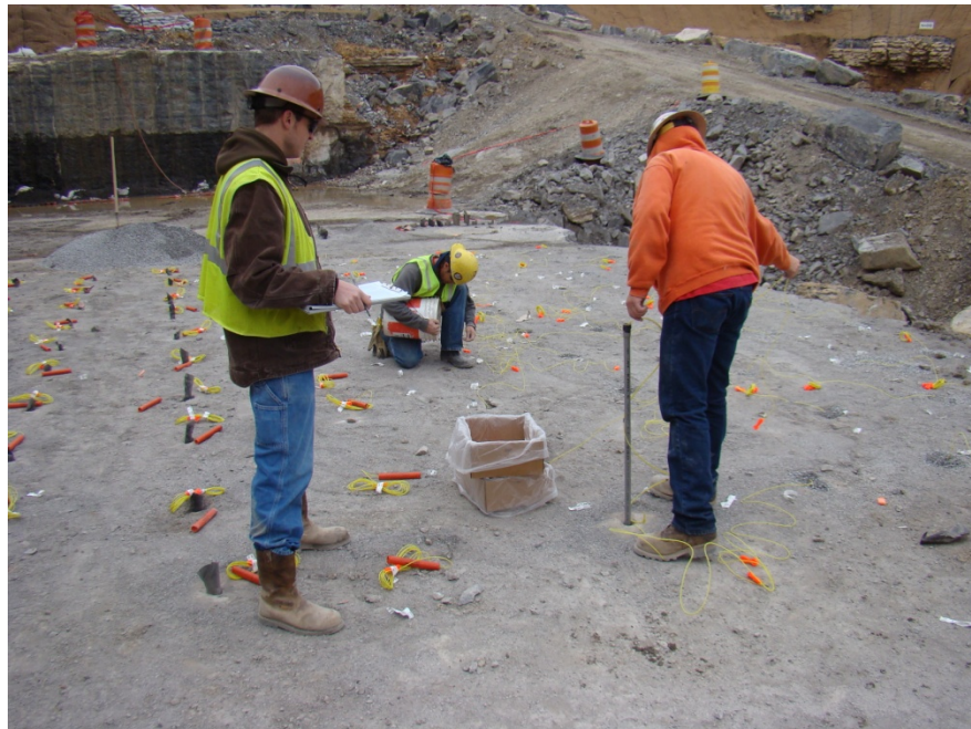
Figure 10-1. Blaster Keeping Records While Loading Shot.
