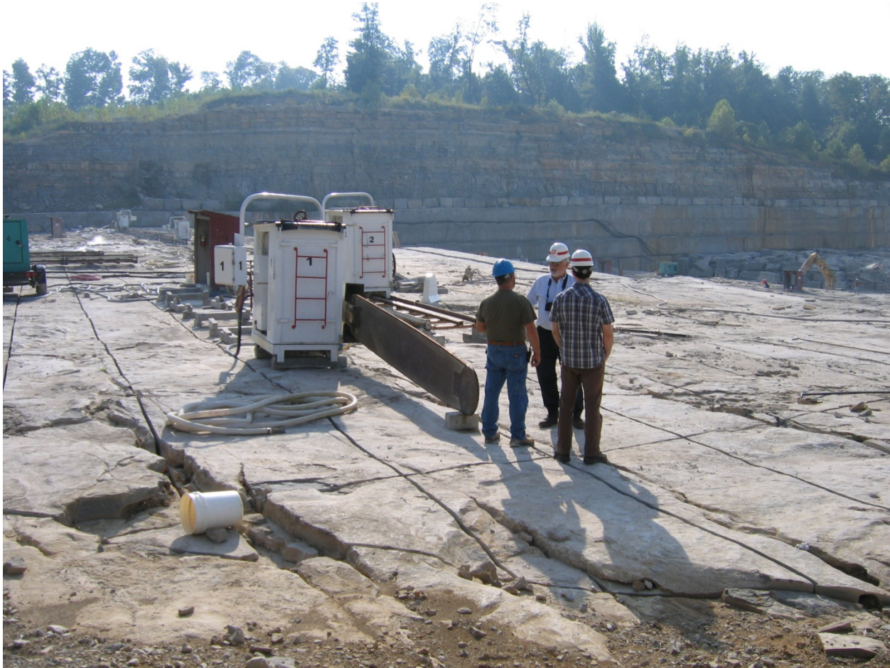
Figure 6-20. Sawing Oolitic Limestone as an Alternative to Blasting.
