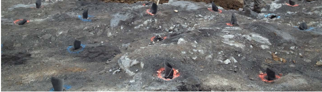
Figure 1-2. Empty Boreholes on a Regularly Spaced Pattern.
