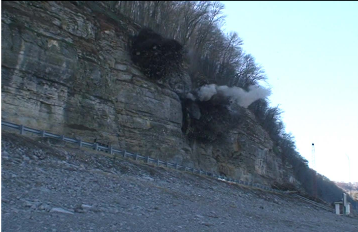
Figure 6-16. Trim Blasting to Remove Unstable Boulders from a Rock Slope.
