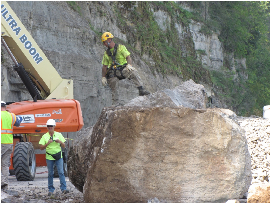
Figure 6-22. Boulder Removed from Slope Using Airbags Shown in Fig 6-21.
