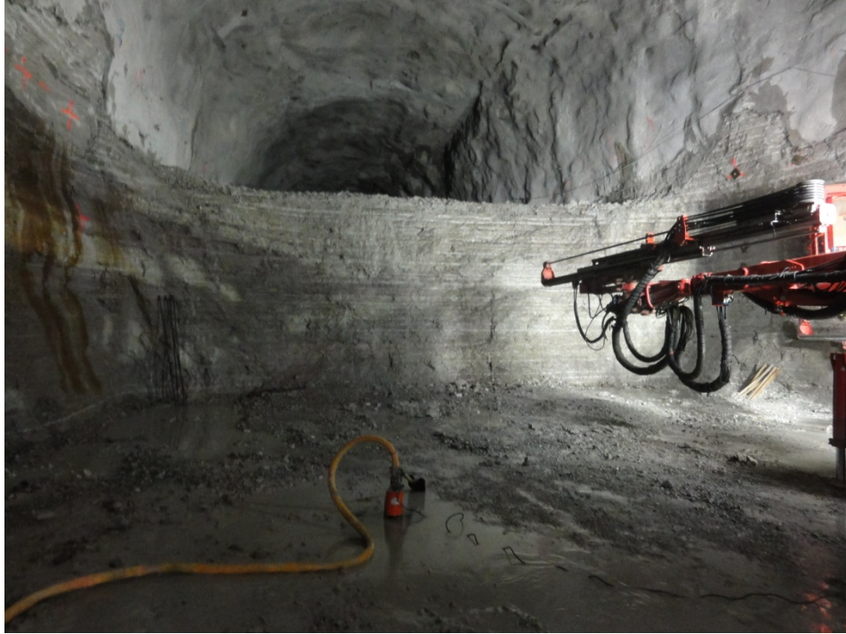
Figure 5-54. Photo of Heading and Bench Method in a Tunnel.
