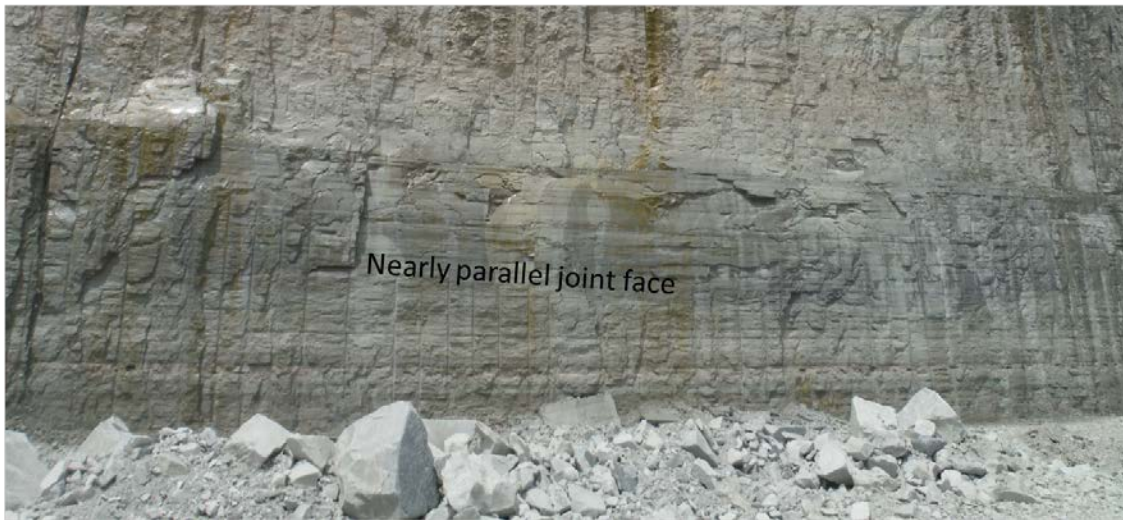
Figure 6-12. Successful Presplit Rock Face with a Nearly Parallel Intersecting Joint. Rock Was Removed Back to Joint Face and No Half Casts Are Visible at Joint Face.
