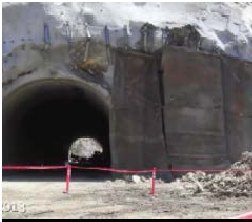
Figure 1-8. Wire Blasting Mats Protects Structures (Courtesy of Mazzella Mats).
