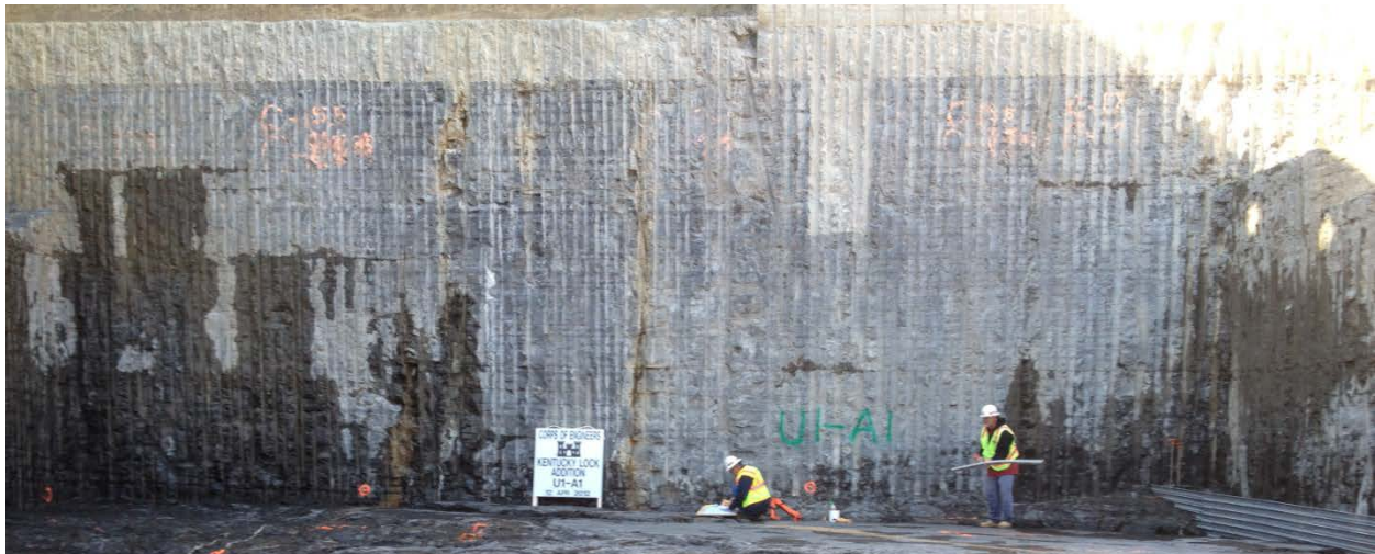
Figure 4-4. Line Drilling for a Lock Construction Project Showing Accurate Drill-Hole Locations.
