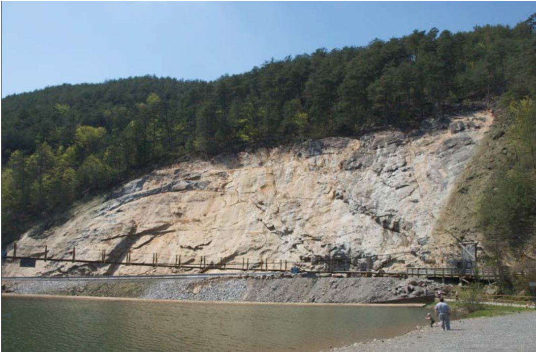
Figure 6-18. View of US64 Slide after Remediation
