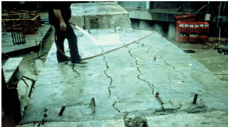
Figure 6-23. Fractures in Rock Created by Rock Splitting Mortar (Courtesy of Da-Mite).
