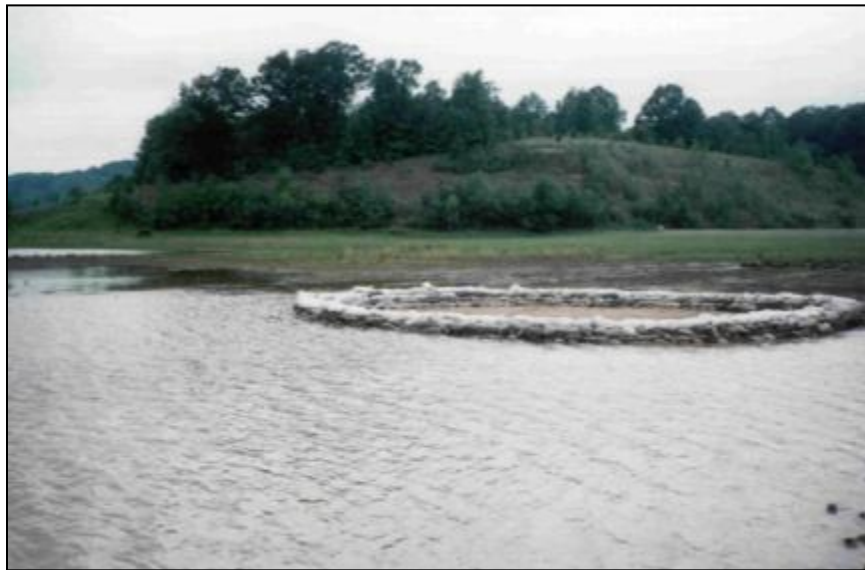
Figure 17-6. Sandbagged dropout sinkhole that developed in an emergency spillway approach channel during a flood at Patoka Dam (Louisville District).
