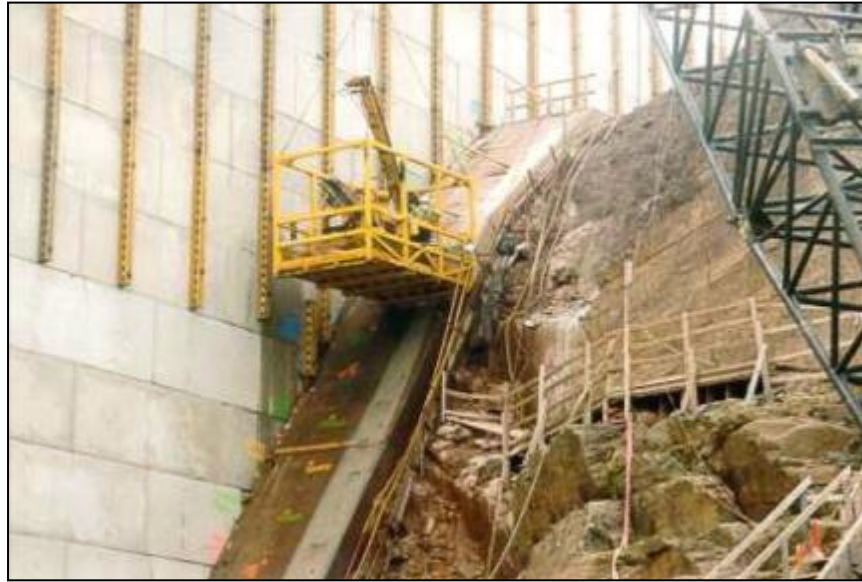
Figure 13-13. Crane-supported drilling platform on a steep abutment.
