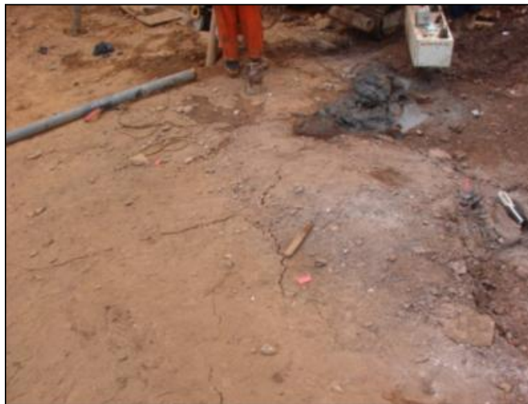
Figure 27-8. Ground surface heave and cracking during compaction grout injection.
