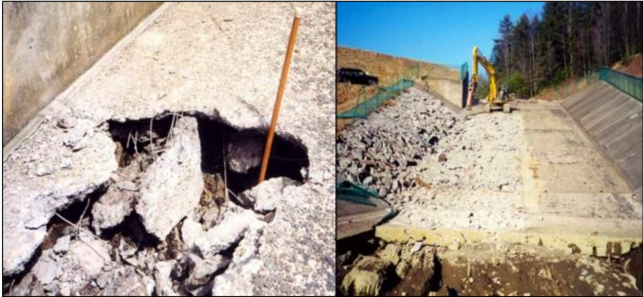
Figure 22-4. Extensive network of large voids beneath a spillway slab, which necessitated demolition and construction of new spillway.
