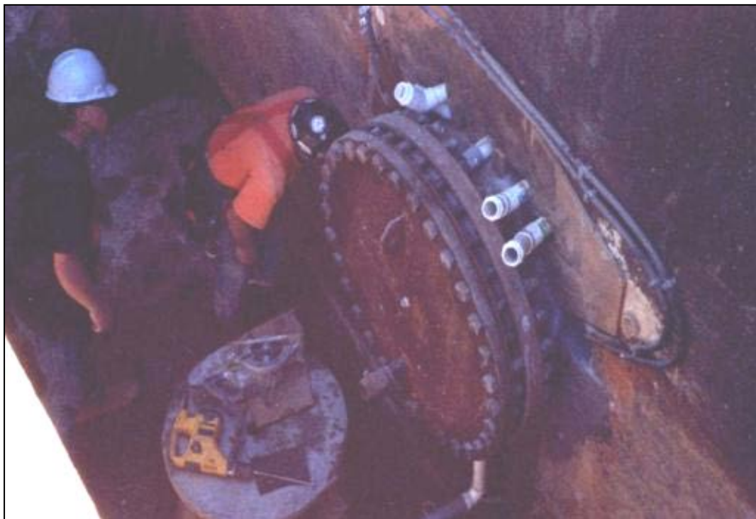
Figure 21-3. Downstream bulkhead with slick lines and air vents at a slip lining project.
