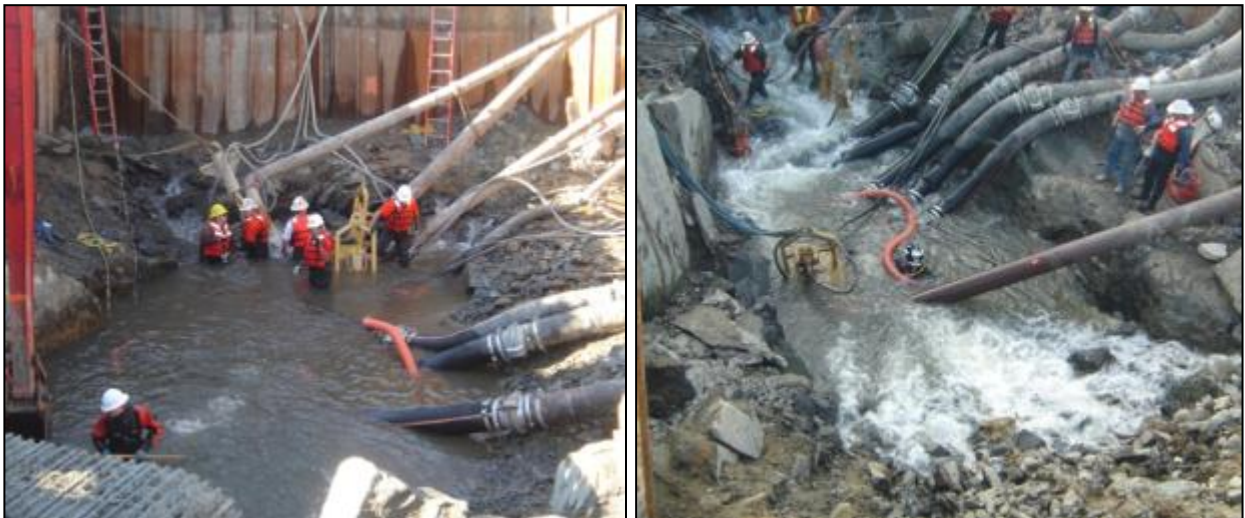
Figure 18-1. Seepage through rock bolt drill holes into a rail tunnel during rehabilitation.
