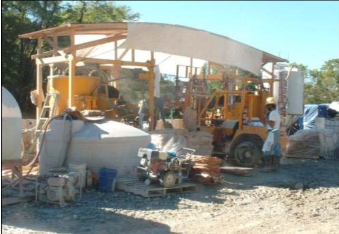
Figure 13-26. Field-constructed shelter over grout mixing station.
