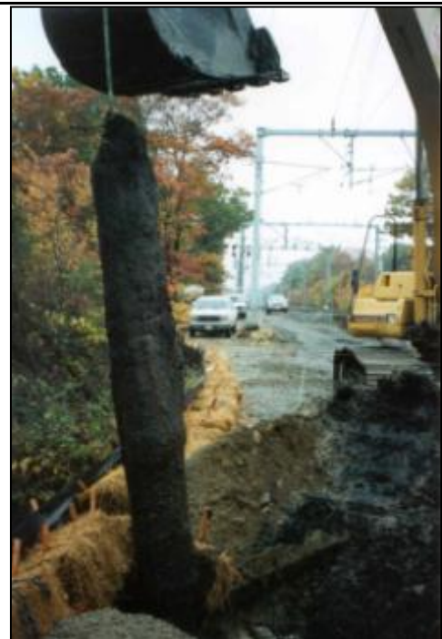
Figure 27-2. Extracted columnar-shaped compaction grout mass.
