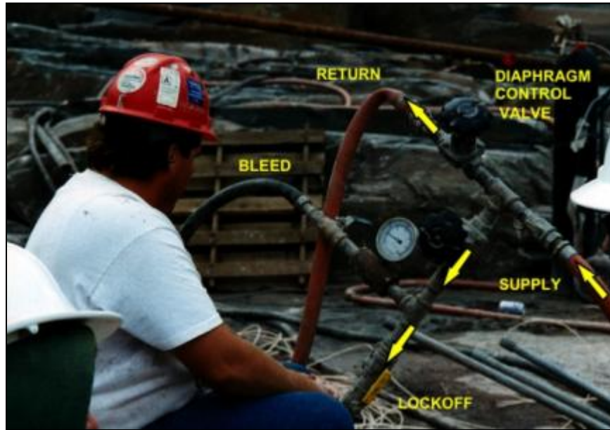
Figure 10-16. Grout header for manual pressure observation and control during HMG injection.
