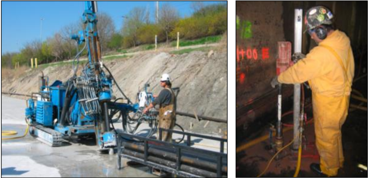
Figure 9-3. Track-mounted and hand-held high-speed rotary drills.
