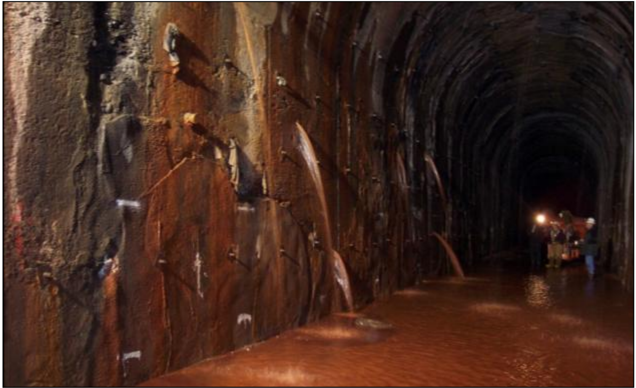
Figure 18-1. Seepage through rock bolt drill holes into a rail tunnel during rehabilitation.
