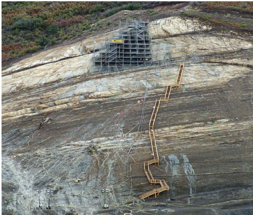
Figure 13-11. Ridges Basin Dam right abutment scaffolding for grouting operations.
