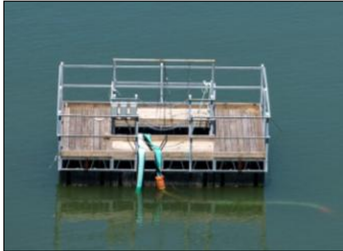
Figure 7-12. Floating water intake for a grouting project during a flood at Mississinewa Dam, IN.
