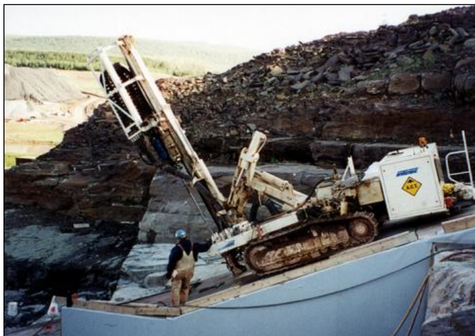
Figure 13-12. Drilling rig operating on an inclined concrete platform.
