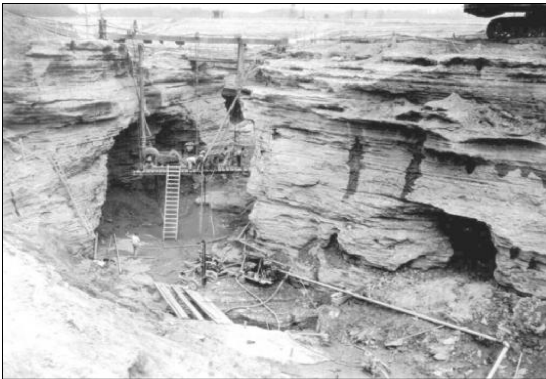
Figure 17-24. Foundation treatment of a network of caves and dissolution channels at Wolf Creek Dam as part of original construction (Nashville District).
