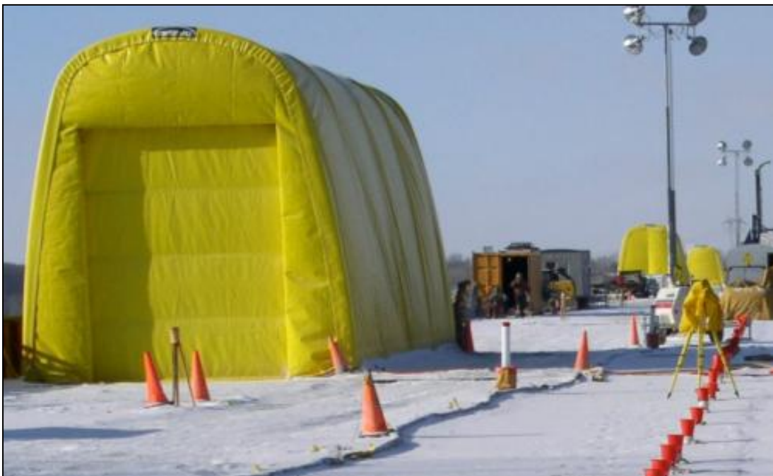
Figure 13-27. Fully enclosed and heated prefabricated shelter for materials storage and mixing.
