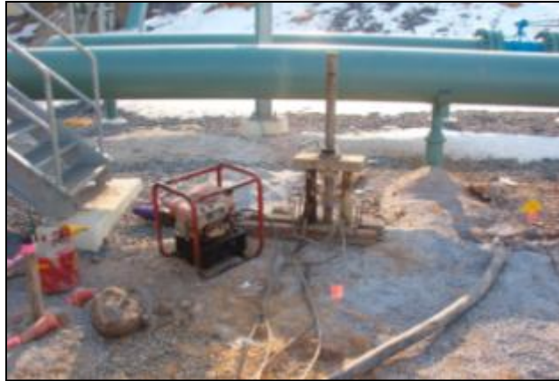
Figure 27-6. Casing withdrawal using extraction jacks.
