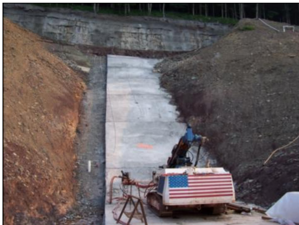
Figure 13-17. Smooth-surface grout cap used on a steep, ledgy, and broken rock surface.
