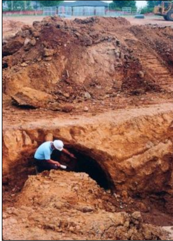
Figure 17-5. Soil arch in an incipient dropout sinkhole in cohesive soil exposed during excavation in Hershey, PA. No surface expression of void was visible. Before excavation, the surface had been proof-rolled with loaded scrapers and compacted. The site had approximately 35 sinkholes with surface expressions.
