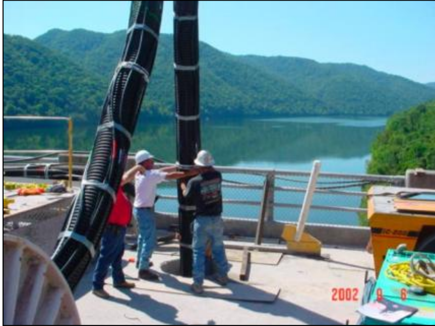
Figure 23-7. Corrugated duct being inserted into the prepared anchor hole at Bluestone Dam, WV (Huntington District). The numerous external tremie tubes are clearly visible.
