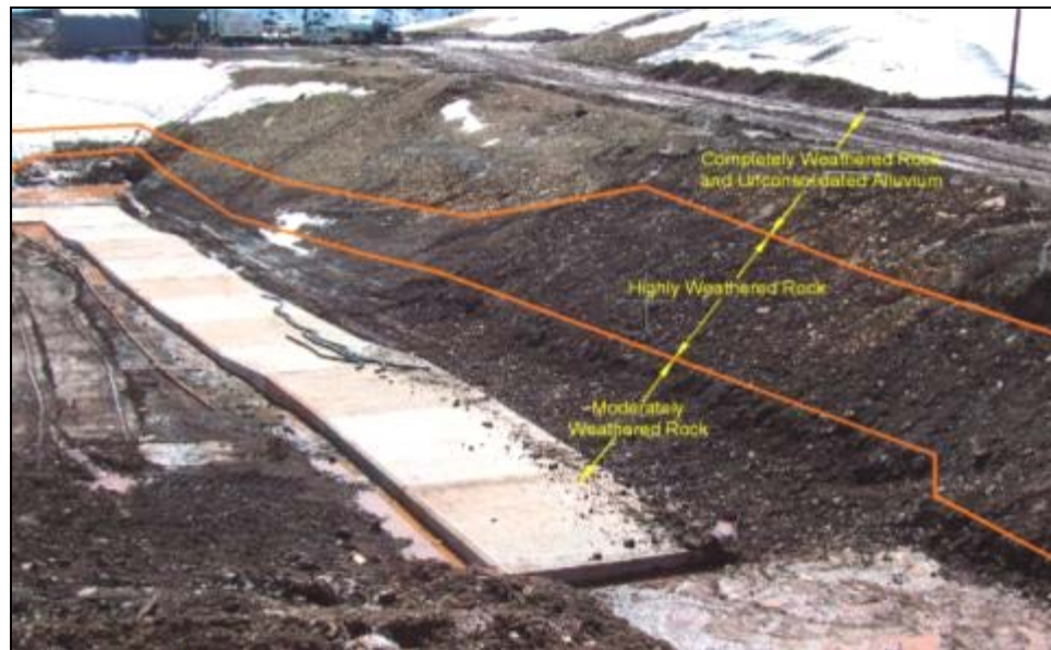
Figure 4-3. Geologic profile in sedimentary rock valley, Lyman Run Dam, PA.
