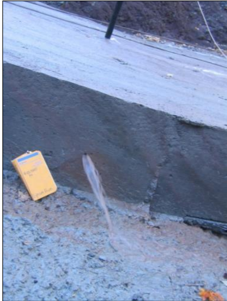
Figure 13-10. Porous grout cap requiring chemical grouting.
