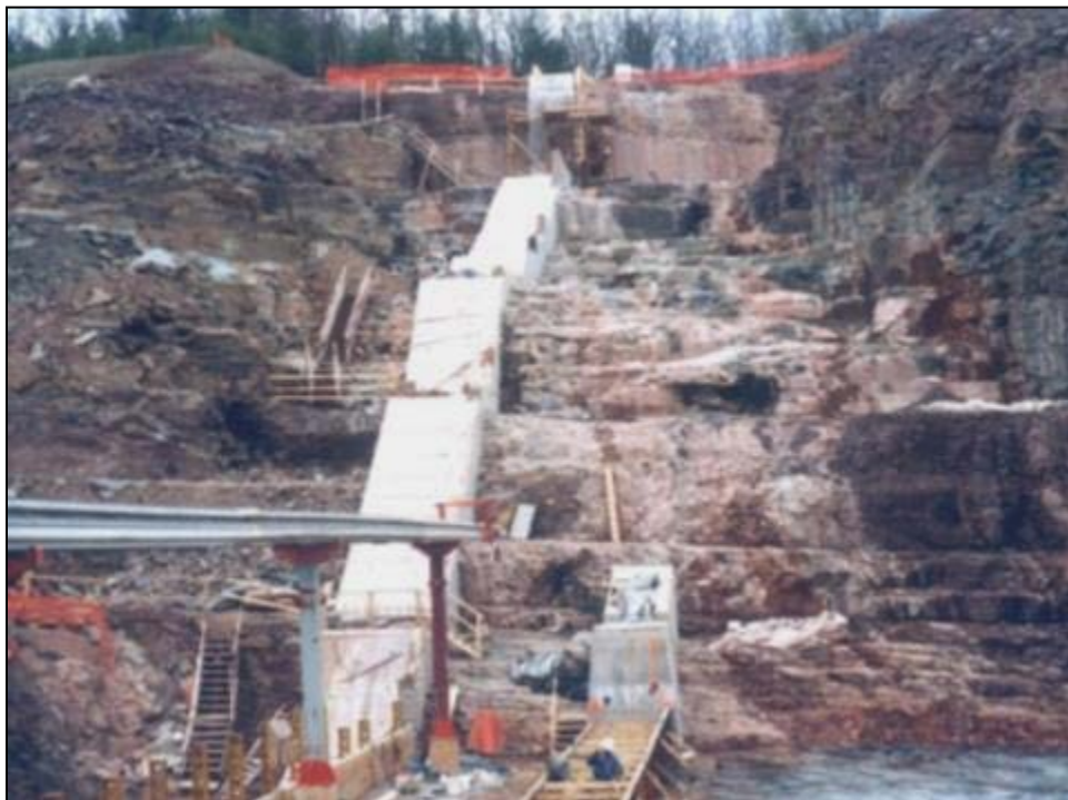
Figure 13-16. Inclined and stepped surface grout cap on a rough, ledgy abutment of a concrete dam foundation.
