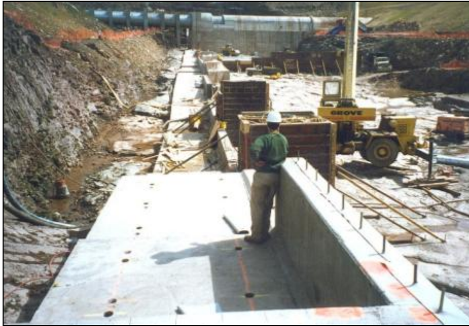
Figure 13-19. Plinth allowing grouting (on left) to be concurrent with RCC dam construction (on right).
