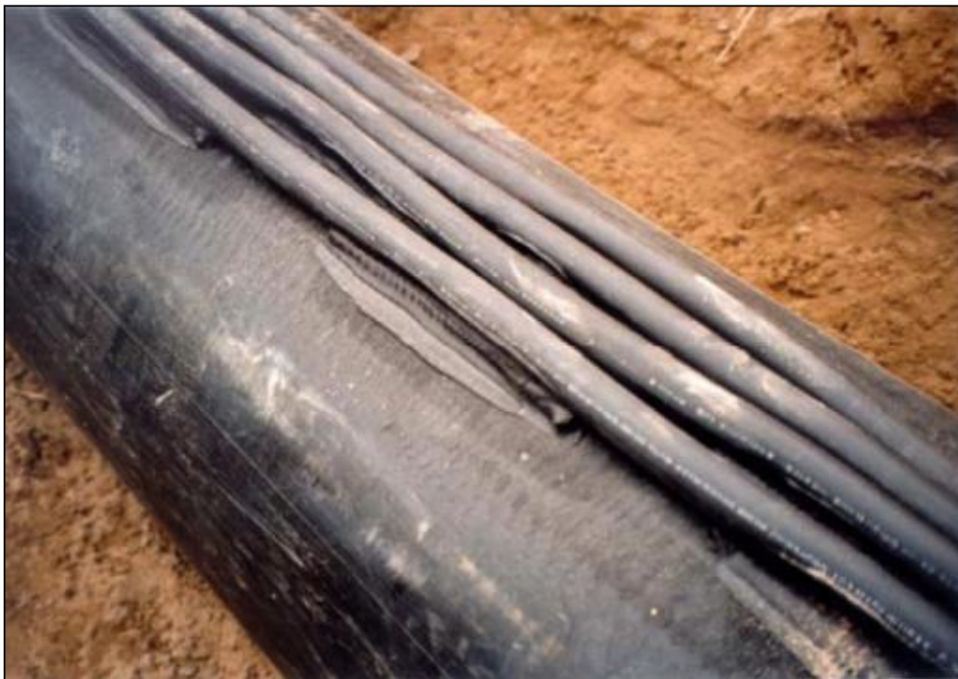
Figure 21-2. Grout pipe slick lines extrusion welded at the crown of an HDPE liner.
