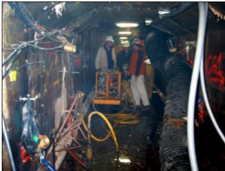
Figure 13-24. Remedial grout injection. Note the crowded conditions in this 9-ft-wide space.
