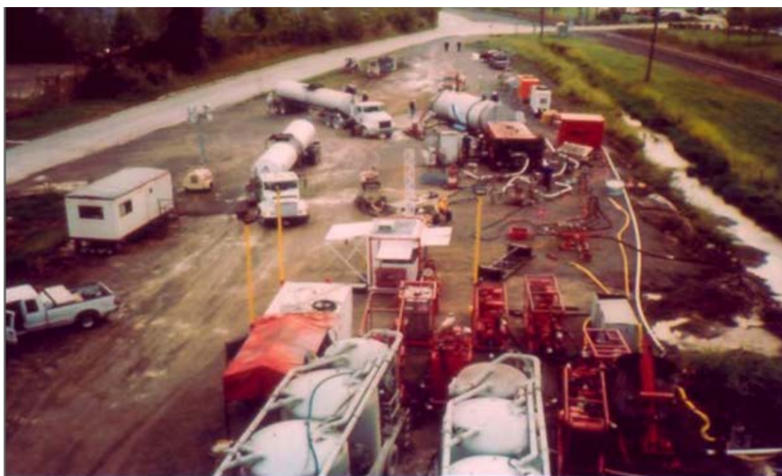
Figure 11-4. Bitumen injection project with heated holding tanks and pumps (foreground), bitumen transport trucks, and injection system (background). Note the high concentration of equipment on this small site.
