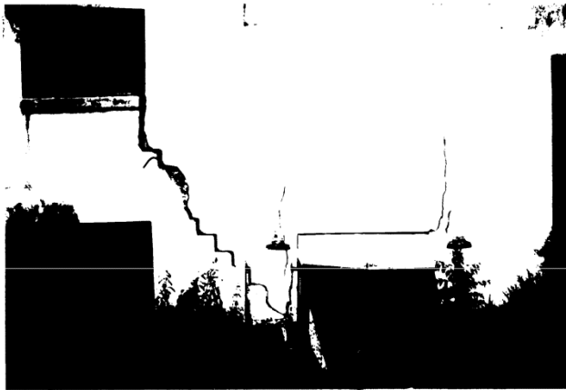
b. Diagonal and vertical cracks
