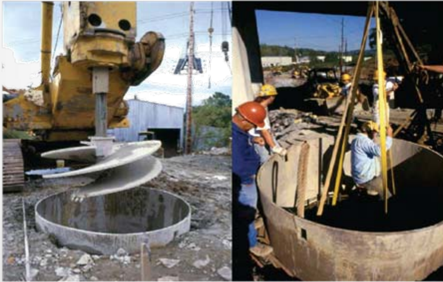
Figure 4-6 Drilling into Rock through a Cased Hole
