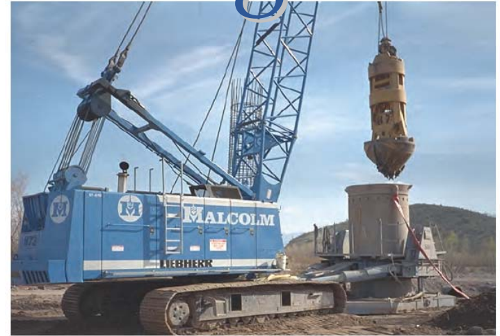
Figure 4-9 Oscillator Rig Used to Advance Segmental Casing Ahead of the Excavation
