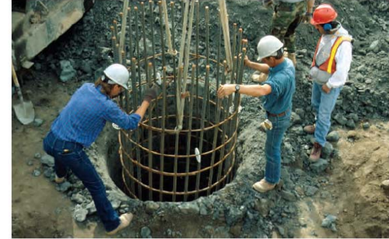
Figure 1-10 Construction of Drilled Shaft in Dry, Cohesive Soils
