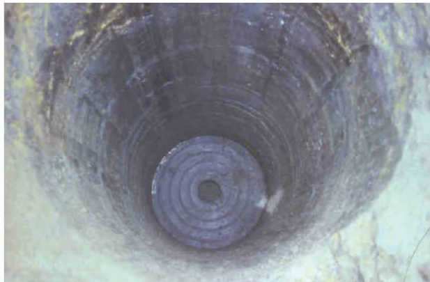
Figure 4-1 Dry Hole in Stable Soil
