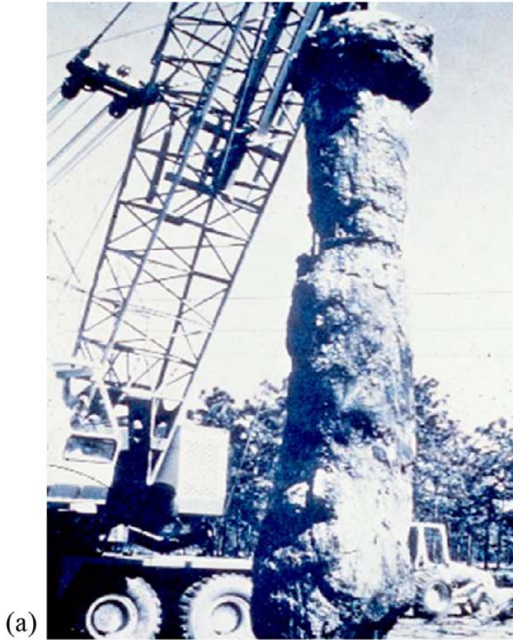
Figure 9-57. Photographs of exhumed shafts (a) shaft where excavation was not adequately cleaned, (b) shaft where excavation was properly cleaned (FHWA, 2002d).
