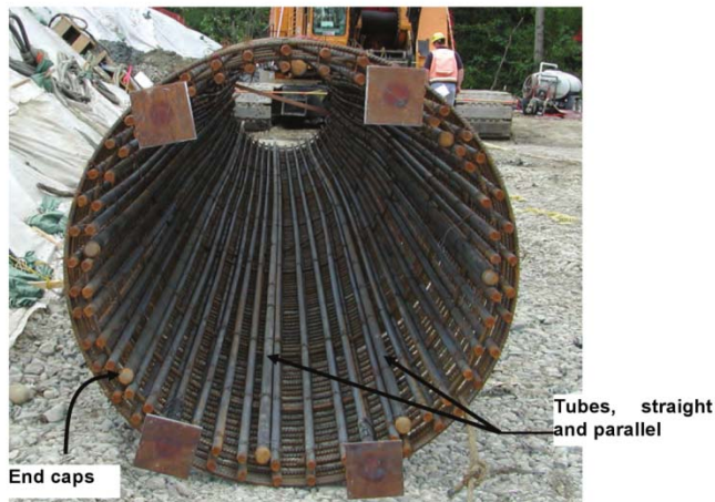
Figure 20-3 Reinforcing Cage with Steel Access Tubes for CSL Testing
