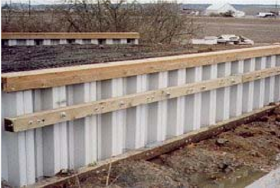
Anchored sheet pile walls
