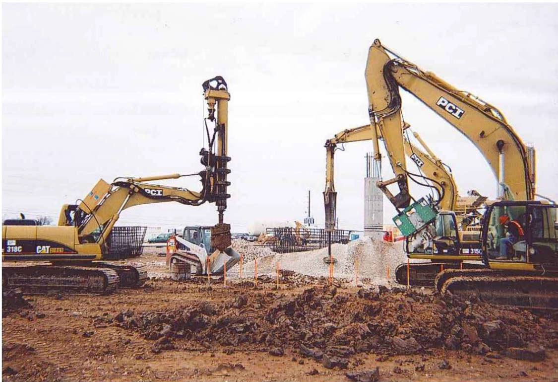
Figure 5-28. Rammed aggregate pier installation.
