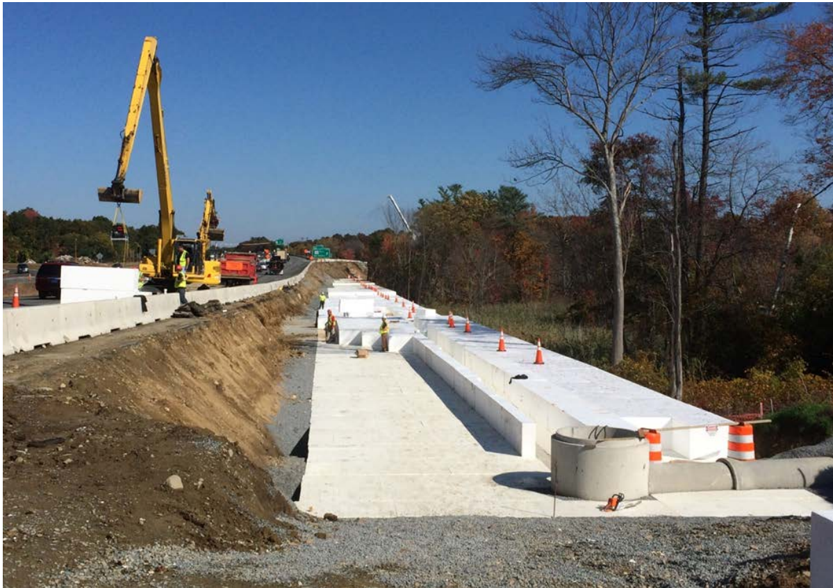
Figure 3-12. Whittier Bridge EPS block placement on embankment widening.
