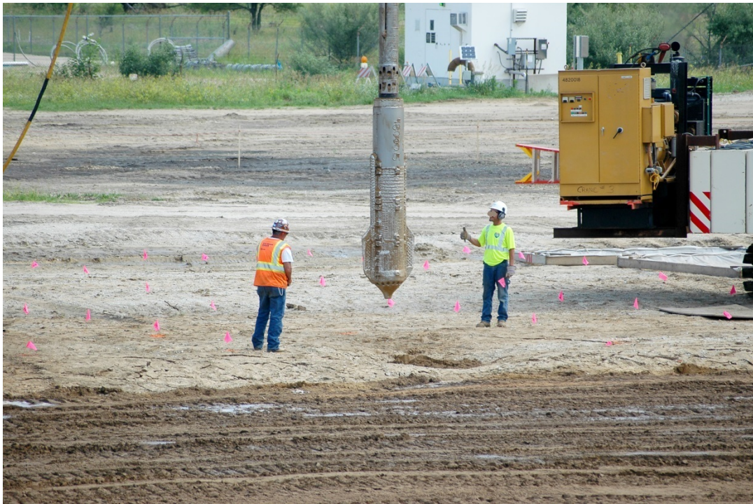
Figure 4-29. High-powered, probe-type vibrator utilized in vibro-compaction.
