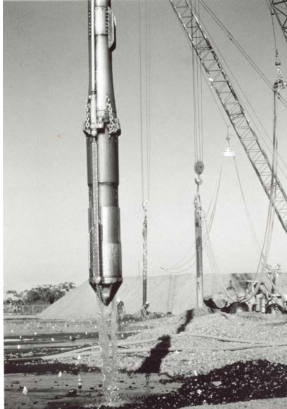
Figure 5-4. Suspended vibrator.
