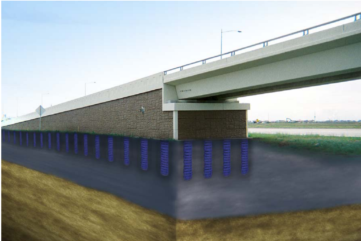
Figure 5-29. Completed MSE wall supported on rammed aggregate piers.
