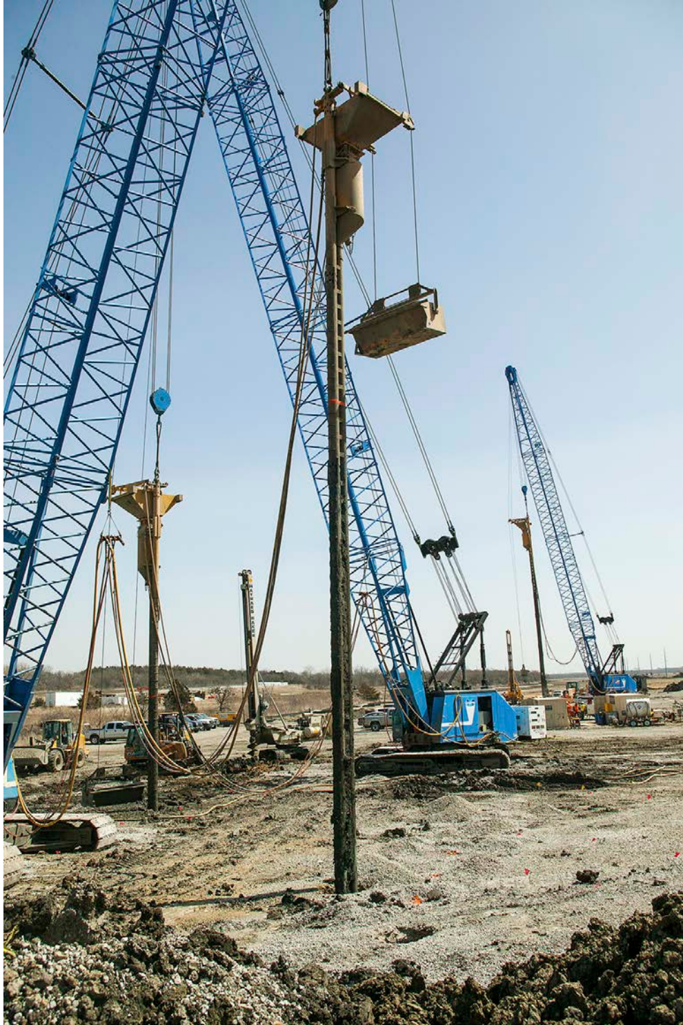
Figure 5-7. Stone column dry bottom feed rig.
