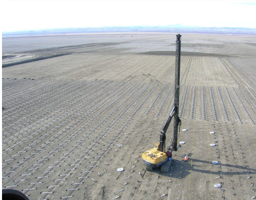
Courtesy Menard Group USA Figure 2-6. Strip drains.
