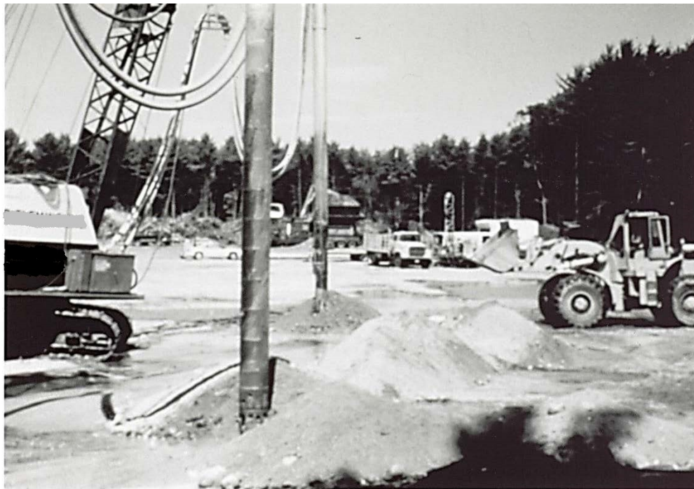
Figure 4-31. Vibrator suspended from a conventional crane.
