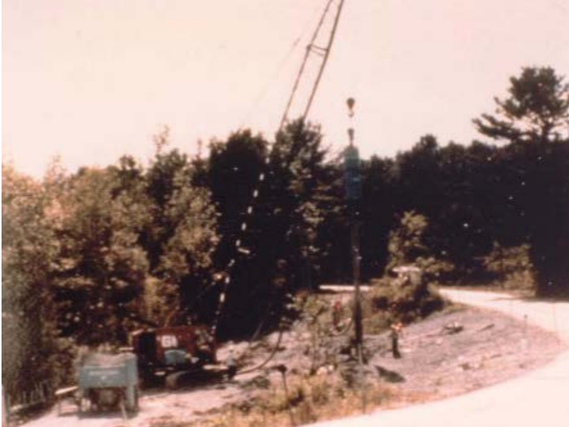
Figure 5-30. Stone column installation.
