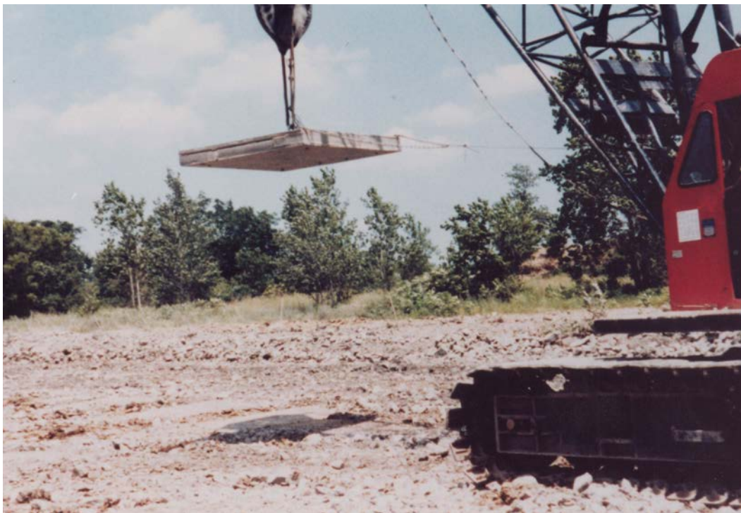
Figure 4-14. Tamper with low contact pressure for ironing pass.
