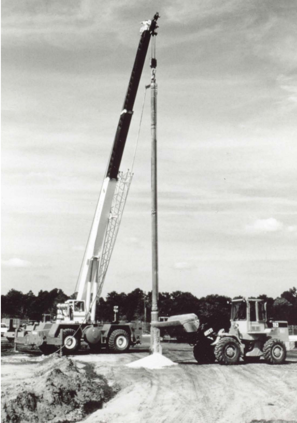
Figure 5-6. Truck mounted crane utilized for top feed vibro-replacement.
