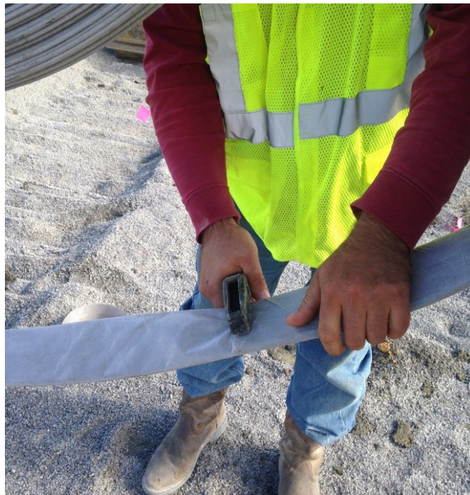
Figure 2-5. Typical prefabricated vertical drain splicing procedure: inserting the drain core within the jacket to maintain continuity (top), stapling the drain splice (bottom).
