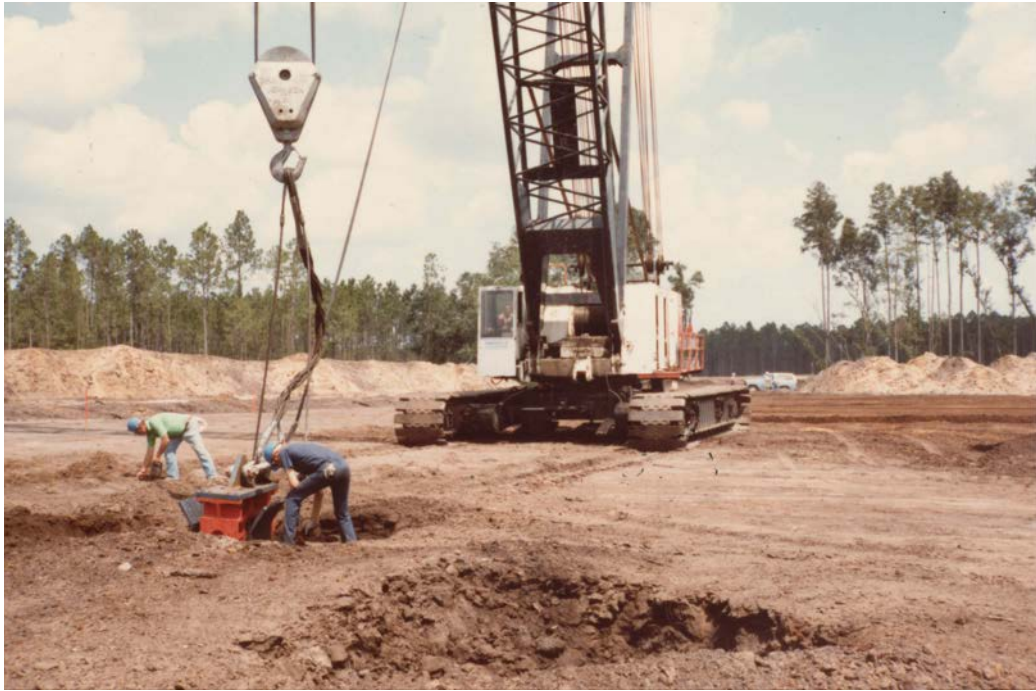
Figure 4-19. Multiple part line used to lift 64 kip tamper (below grade in photo).
