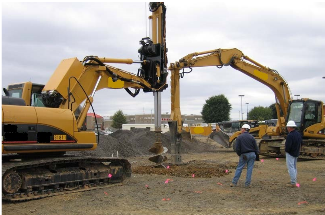
Figure 5-15. Replacement method, rammed aggregate pier with predrilling.
