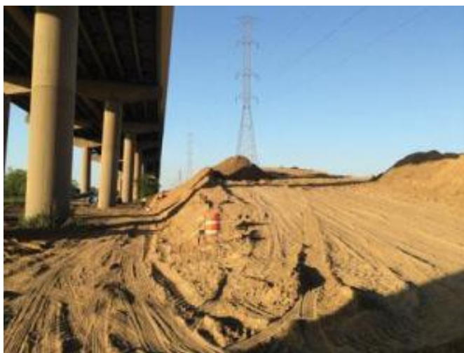
Figure A-6: Tilting bridge piers and adjacent soil stockpile (O'Shea, 2015)
