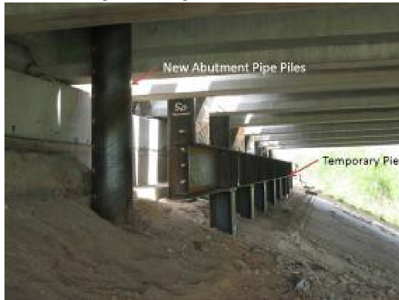
Figure A-18: Repairs and New Foundations (DeStephen, 2015)
