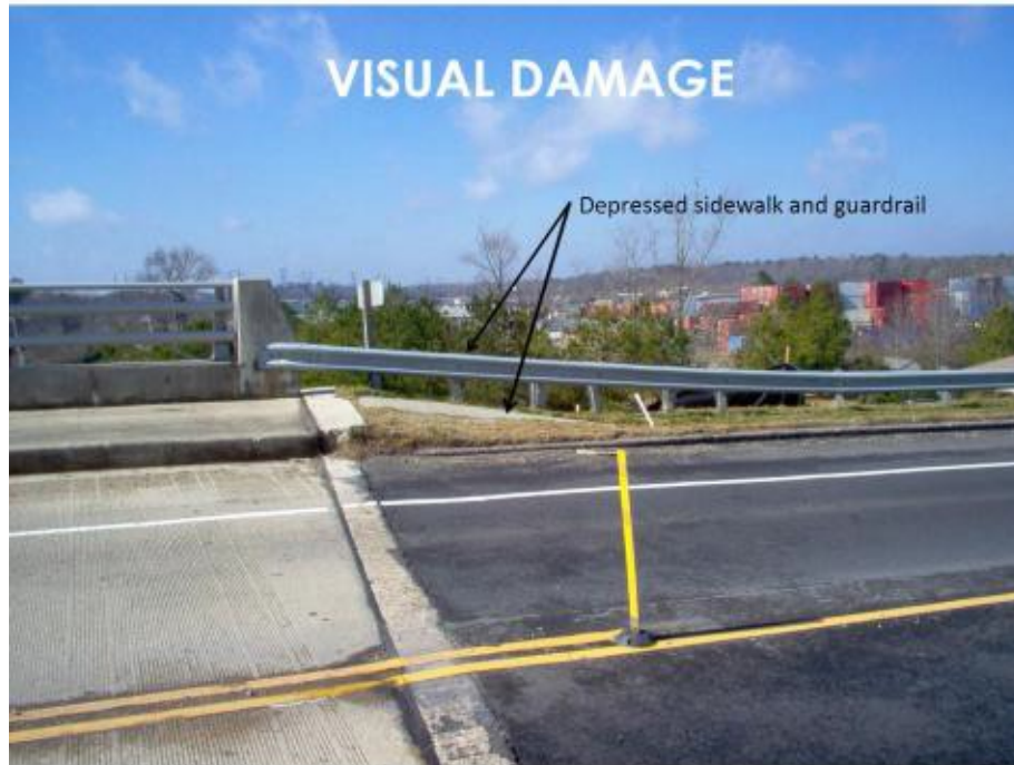
Figure A-16: Damage from Settlements (DeStephen, 2015)
