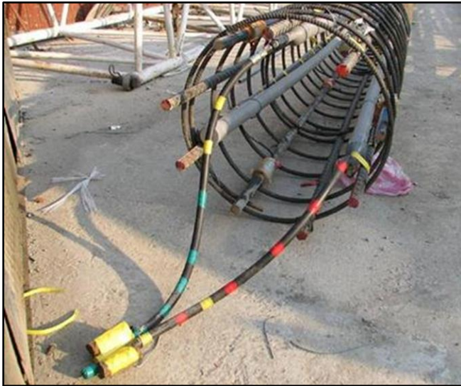
Figure 5.6: Photograph of a sleeve-port system constructed using flexible hoses (courtesy of Dr. H.H. Hsieh).
