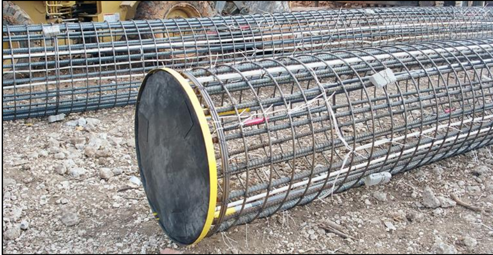
Figure 5.9: Flat-jack post-grouting device on a 4-ft diameter shaft (photo courtesy of Applied Foundation Testing).
