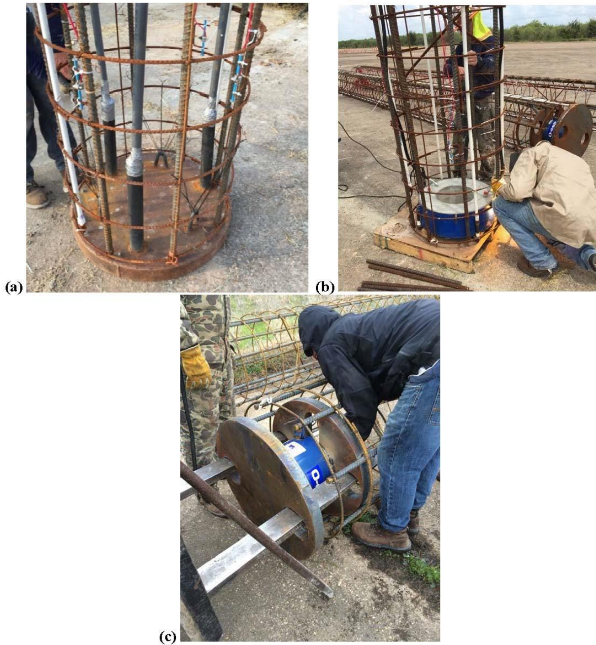
Figure 10.3: Bi-directional loading devices: (a) flat jack, (b) RIM Cell, and (c) O-Cell.
