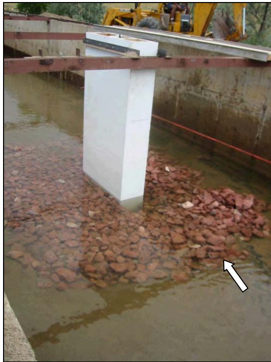
Figure 11.14. Riprap armor over geotextile containers.
