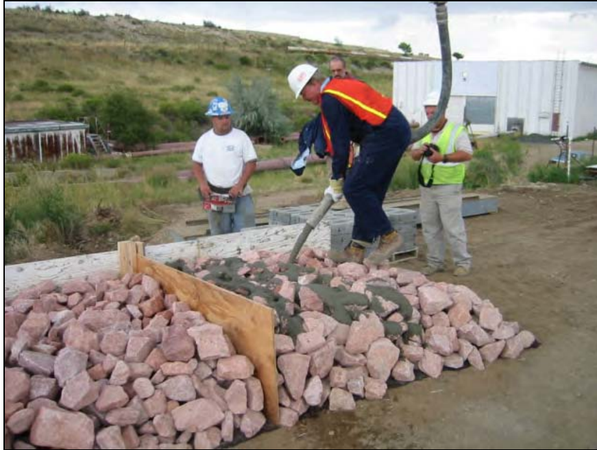
Figure 12.8. Preliminary trial grout application in the dry.
