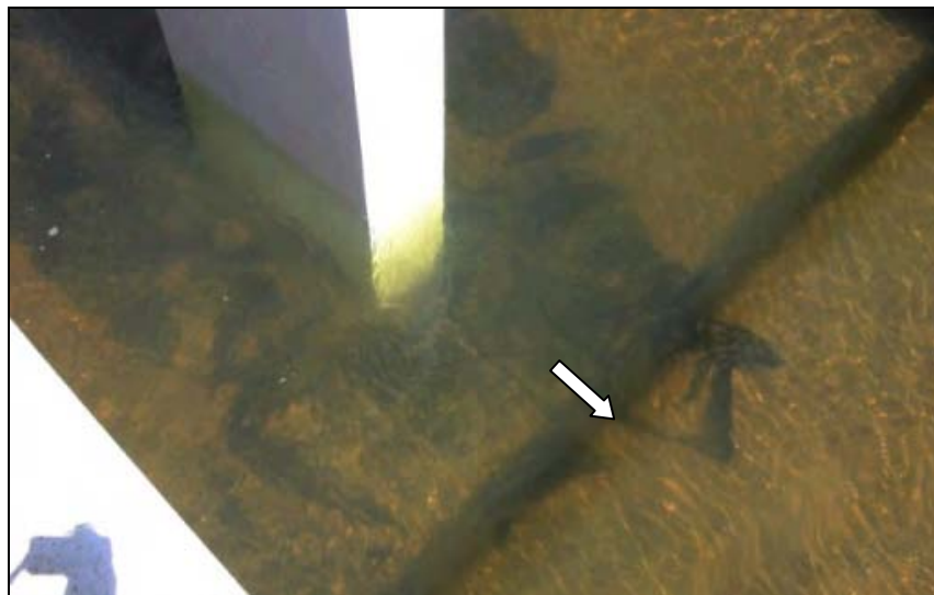
Figure 11.12. Geotextile containers after installation.
