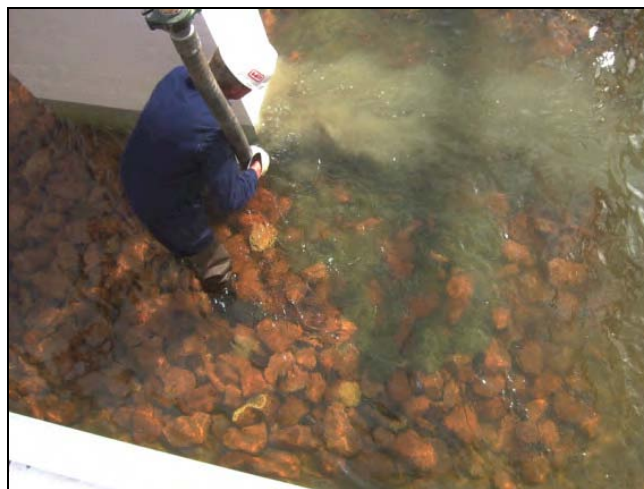
Figure 12.11. Underwater partial grouting of riprap.
