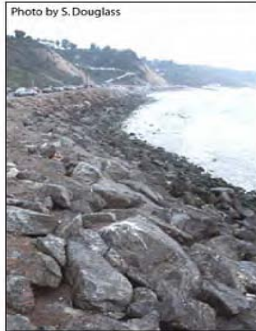
Figure 17.1. Riprap revetment in a wave environment, Pacific Coast Highway, California. (from HEC-25, 2nd Edition)
