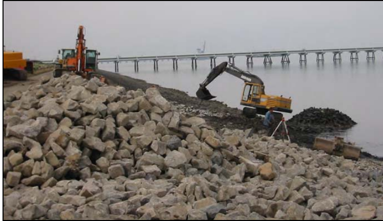
Figure 12.18. Placing riprap with hydraulic excavators.
