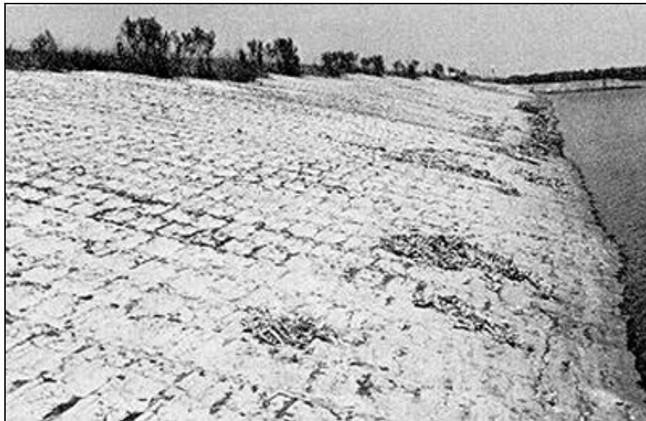
Figure 7.3. Soil cement placed in the plating method parallel to the slope (PCA).
