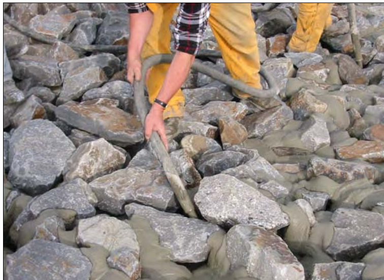
Figure 12.20. Grout placement by hand.
