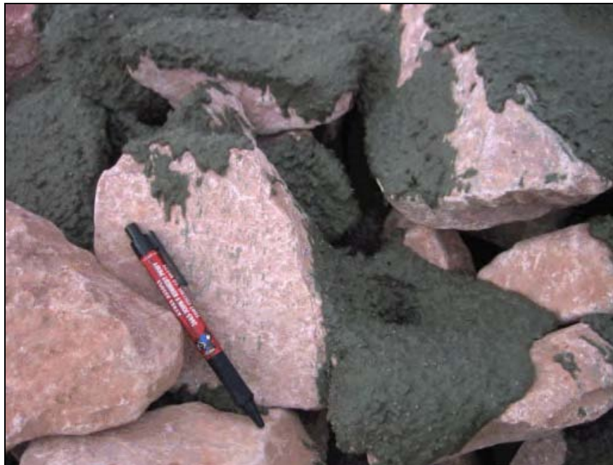
Figure 12.9. Surface of the riprap after partial grouting.
