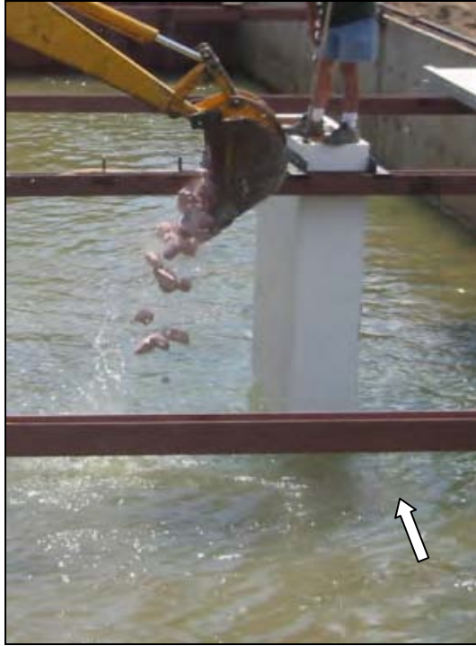
Figure 11.13. Installation of riprap around pier.
