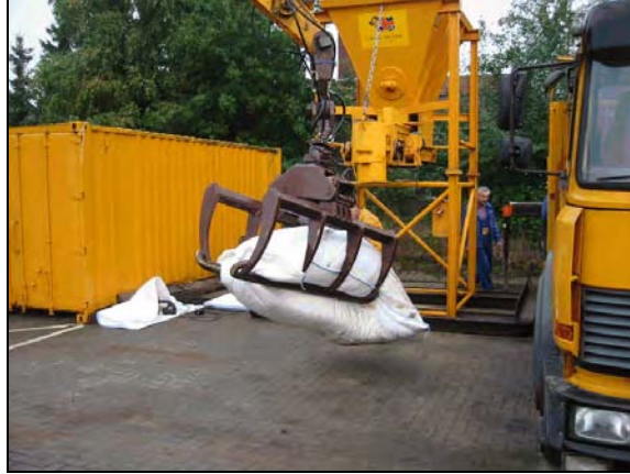
Figure 11.20. Handling a one-tonne sand-filled geotextile container. (photo from NCHRP Project 24-07(2), courtesy Colcrete – Von Essen Inc.)
