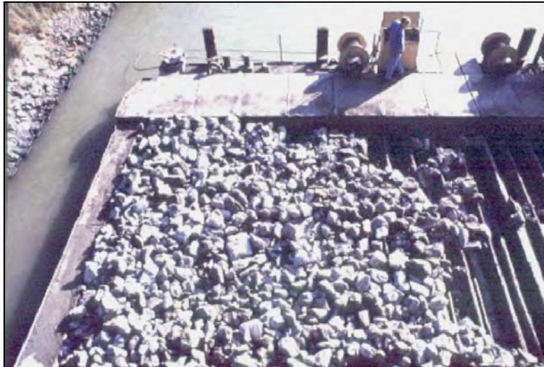
Figure 4.9. Bottom dump pontoon barge used in Germany for placing riprap (TRB 1999).
