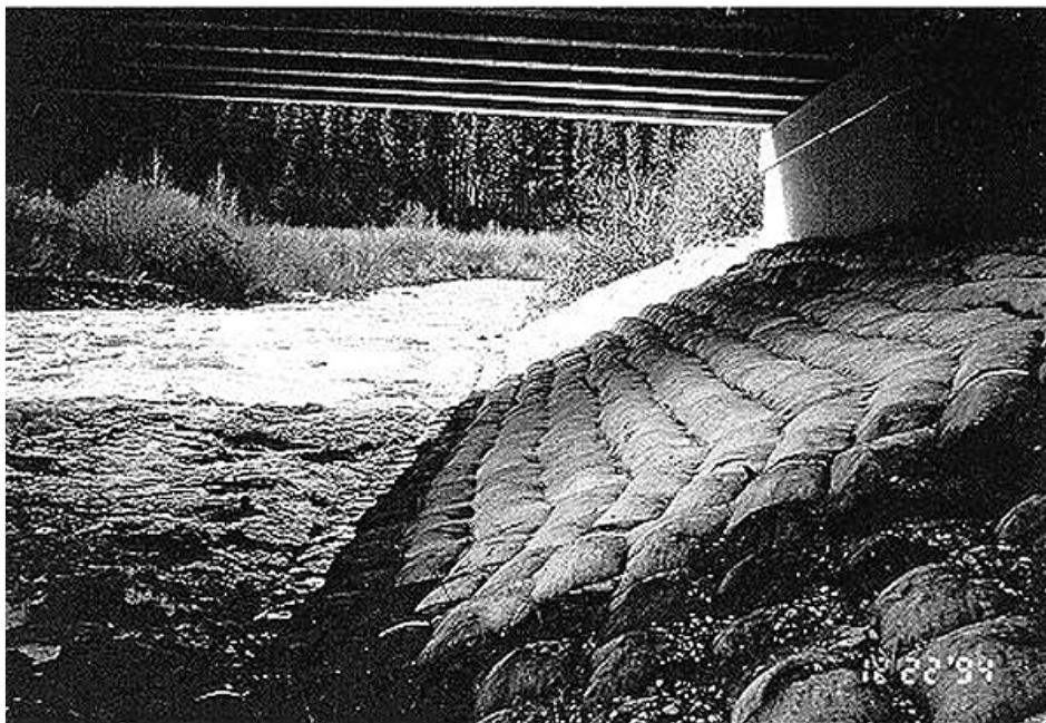
Figure 9.10. ABM underneath Salmon Creek Bridge (ODOT).
