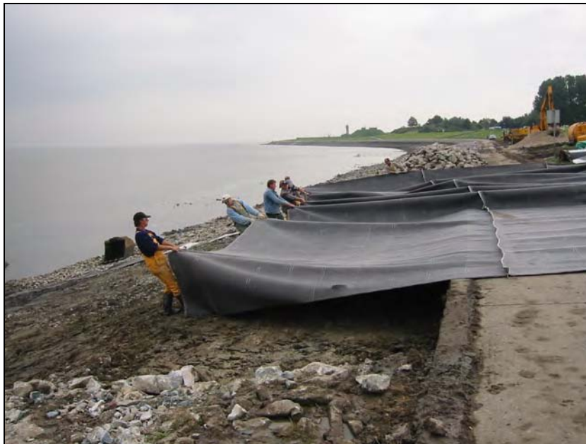
Figure 12.17. Hand placing geotextile prior to placing partially grouted riprap. Note sewn seam.
