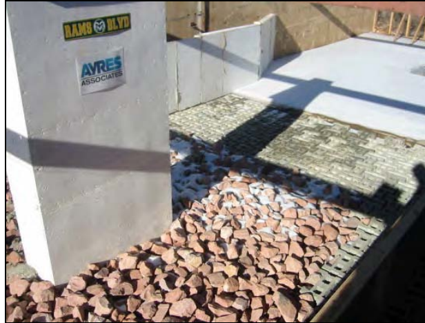
Figure 12.12. Loose riprap, ACB, and contraction wall installation (note loose riprap on the near side of the pier and partially grouted riprap on the far side).
