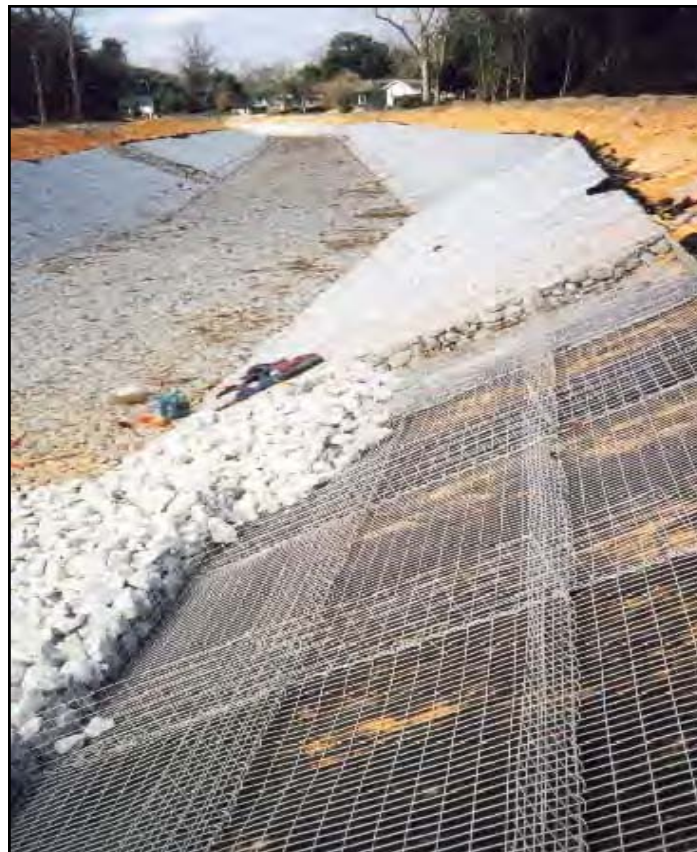
Figure 10.2. Field installation of gabion mattresses on channel bed and banks.
