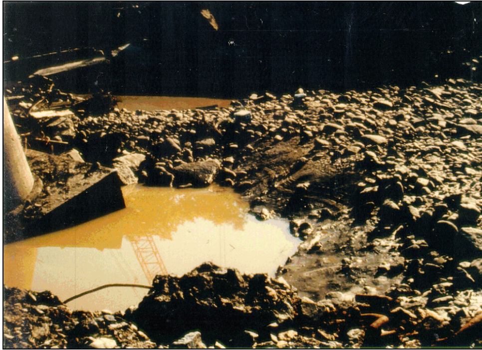
Figure 5.17. Pier scour holes at Schoharie Creek Bridge in 1987. Pier 2 in the foreground with pier 3 in the background.
