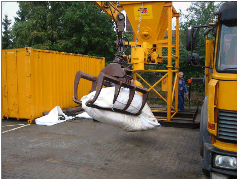
Figure 5.6. Handling a 1.0 metric tonne sand-filled geotextile container. (photo from NCHRP Project 24-07(2), courtesy Colcrete – Von Essen Inc.)
