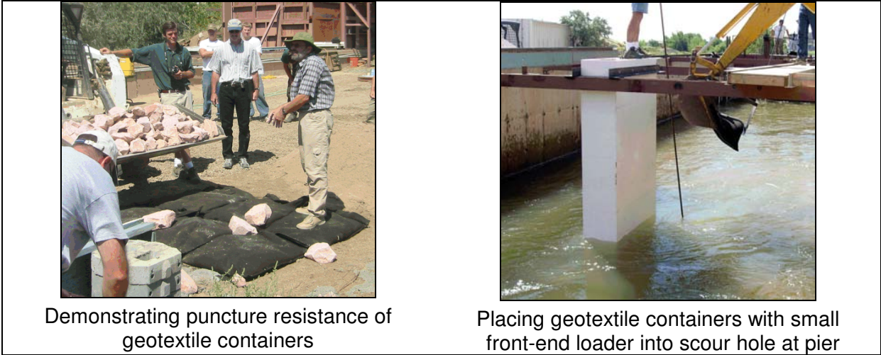
Figure 5.7. Two hundred lb (91 kg) sand-filled geotextile containers, NCHRP Project 24-07(2).
