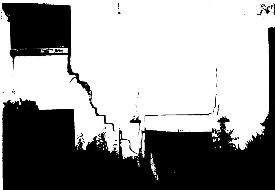
b. Diagonal and vertical cracks
