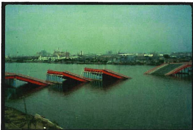
Fig. AIII-7: Collapse of the Showa Bridge (Steinbrugge Collection, Earthquake Engineering Research Center, University of California, Berkeley).
