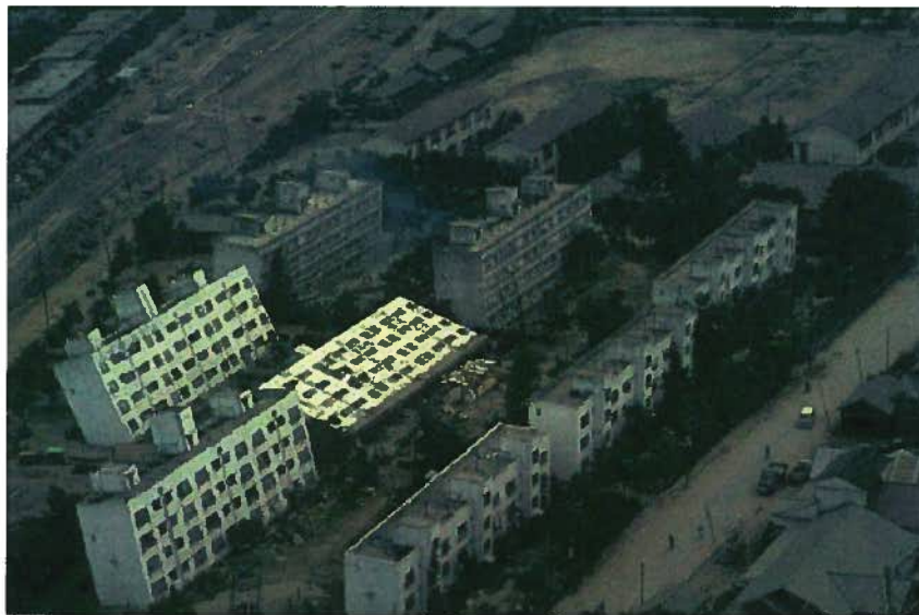
Fig. AIII-6: Liquefaction-induced bearing capacity failures of the Kawagishi-Cho apartment buildings (USGS, from Kramer, 1996).
