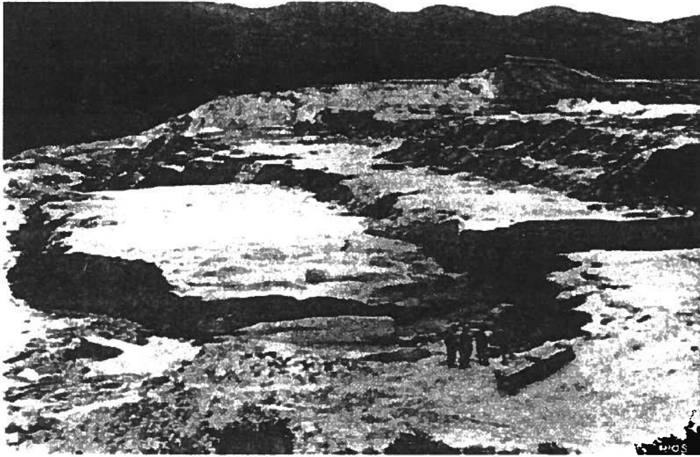
Fig. AIII-2: Photo of the failure zone showing terraces of tailings soils left in place (Troncoso et al. 1993).
