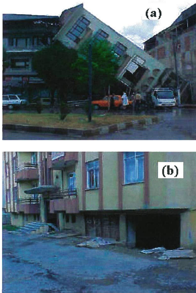
Fig. 3-1: Liquefaction foundation failure, (a) Overturning and (b) settlement of structures resulting from liquefaction of foundation soils in Adapazari, Turkey, 1999 (adapted from Kammerer, 2002).
