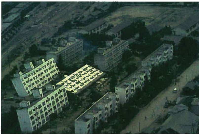
Fig. 3-33: Liquefaction-induced bearing capacity failures of the Kawagishi-Cho apartment buildings (EERC, Un., Cal, Berkeley).
