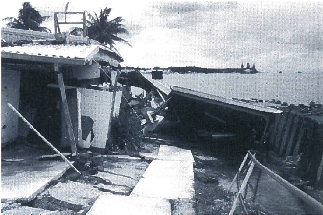
Fig. AIII-18: Damage to Andy's Hut due to liquefaction and lateral spreading (EERI, 1995).
