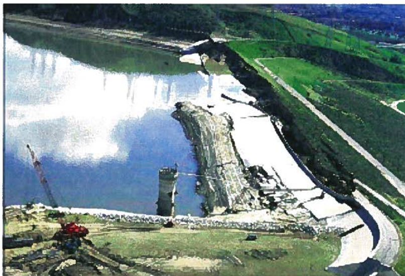
Fig. AIII-10: Flow failure of the upstream slope of the Lower San Fernando dam (Steinbrugge collection; EERC, Univ. of California, photo from Kramer, 1996).
