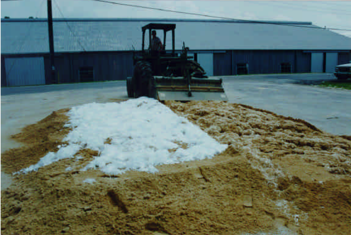
Photo 9. Field mixing of monofilament fibers and concrete sand
