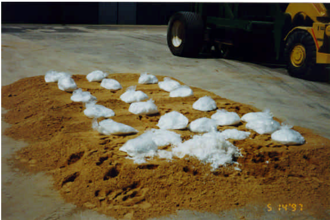
Photo 8. Sand and monofilament fibers prior to mixing in the staging area
