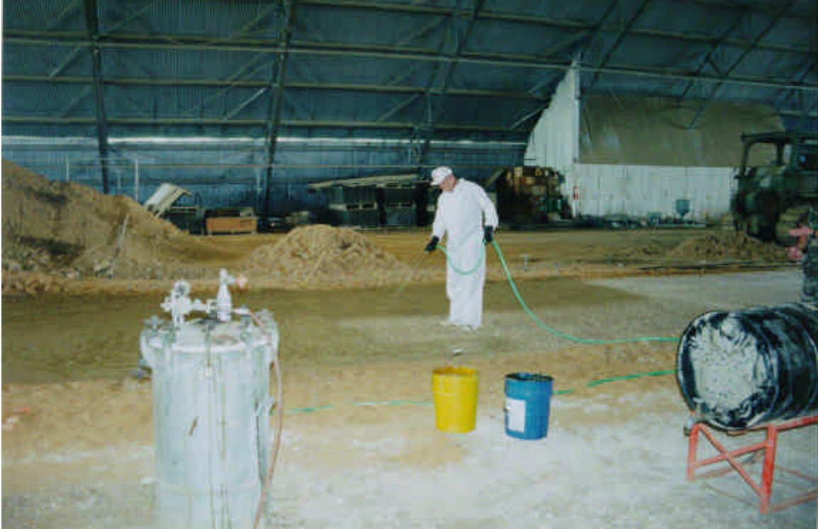
Photo 13. Application of spray-on surfacing at 1 gsy
