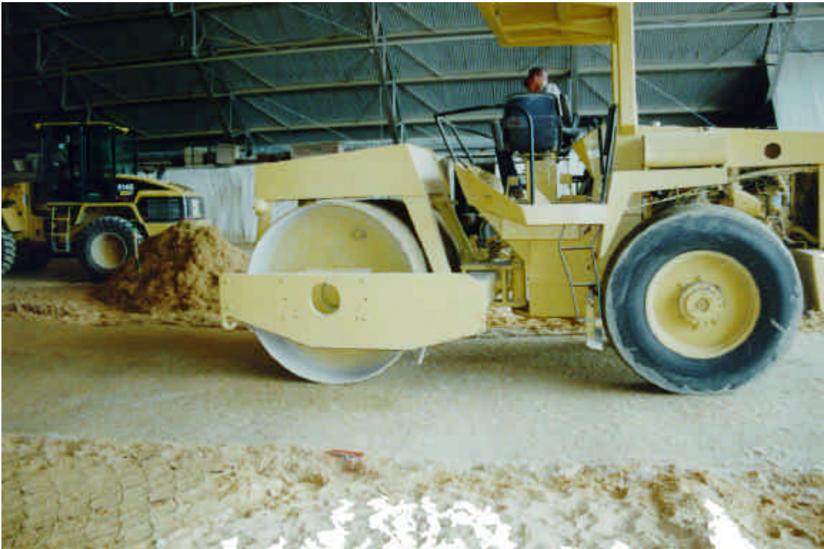
Photo 12. Field compaction of experiment item
