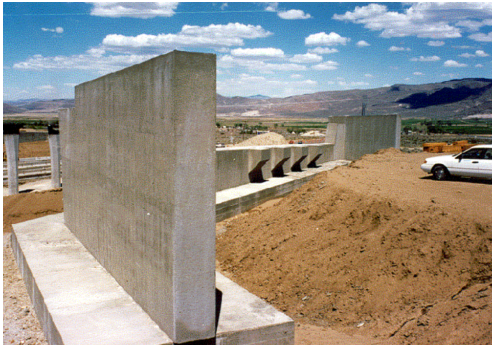
Figure 1: Continuous Foundations (from [Kimmerling (2002)])
