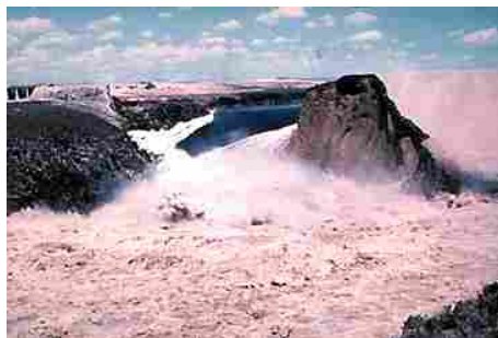
Figure 7.2: Failure of Teton Dam.
