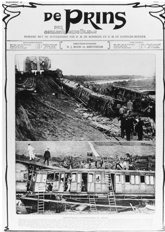
Figure 1.1: Landslide near Weesp, 1918.
