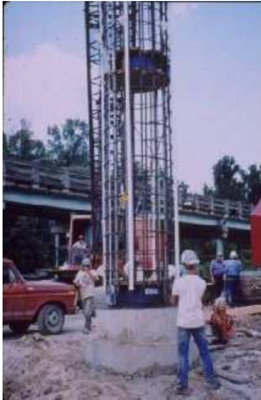
Figure 38, Osterberg Load Cells
