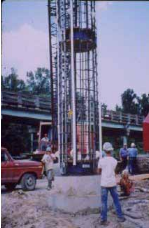
Figure 41, Osterberg Load Cells
