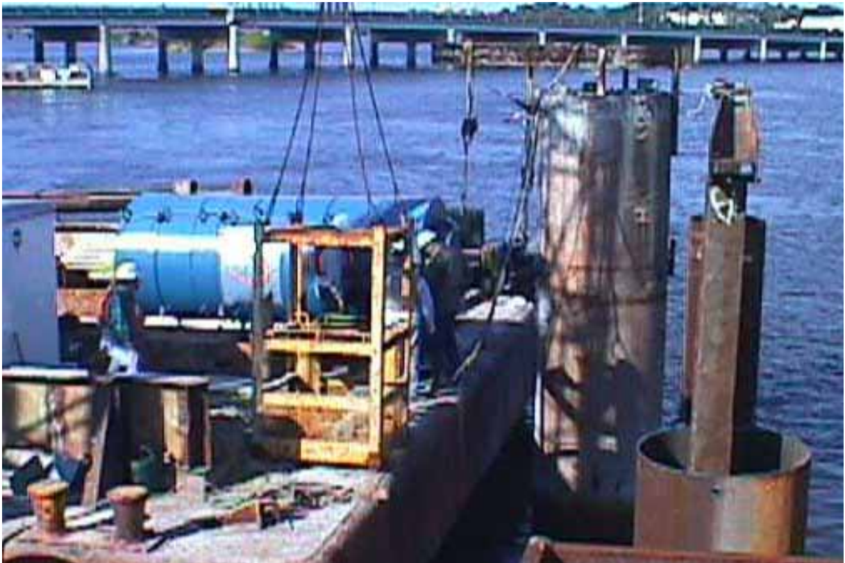
Figure 40, Lateral Static Load Test
