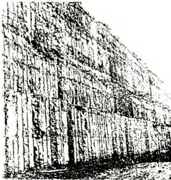
Figure 4.3. Presplit Blasting in Limestone.
