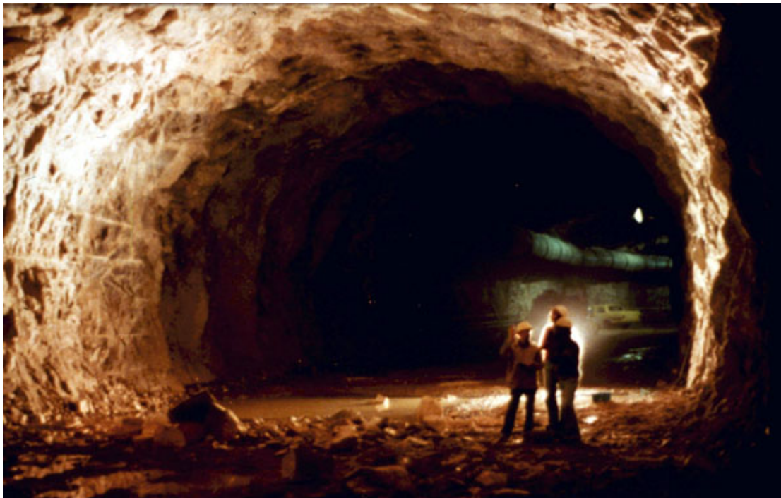
Figure 6.1: The 12 m span 8 m high top heading for the tailrace tunnel was constructed by full-face drill-and-blast and, because of the excellent quality of the massive gneiss, was largely unsupported.
