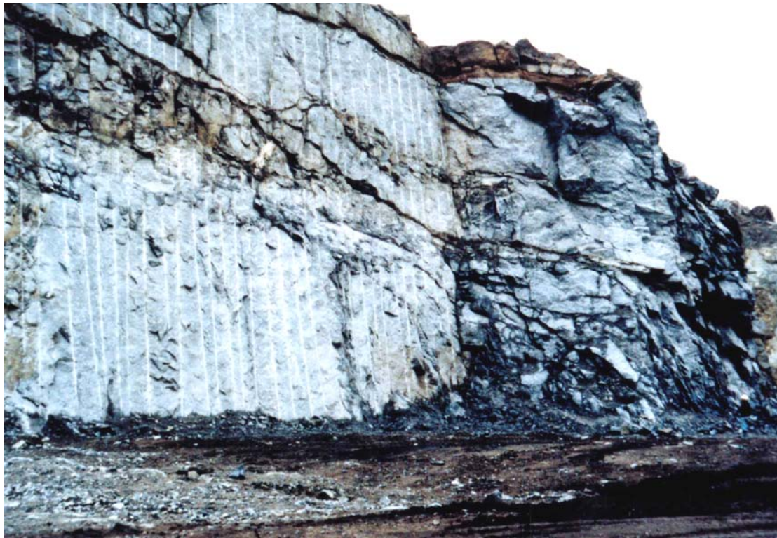
Figure 11.6: Comparison between the results achieved using controlled blasting (on the left) and normal bulk blasting for a surface excavation in gneiss.
