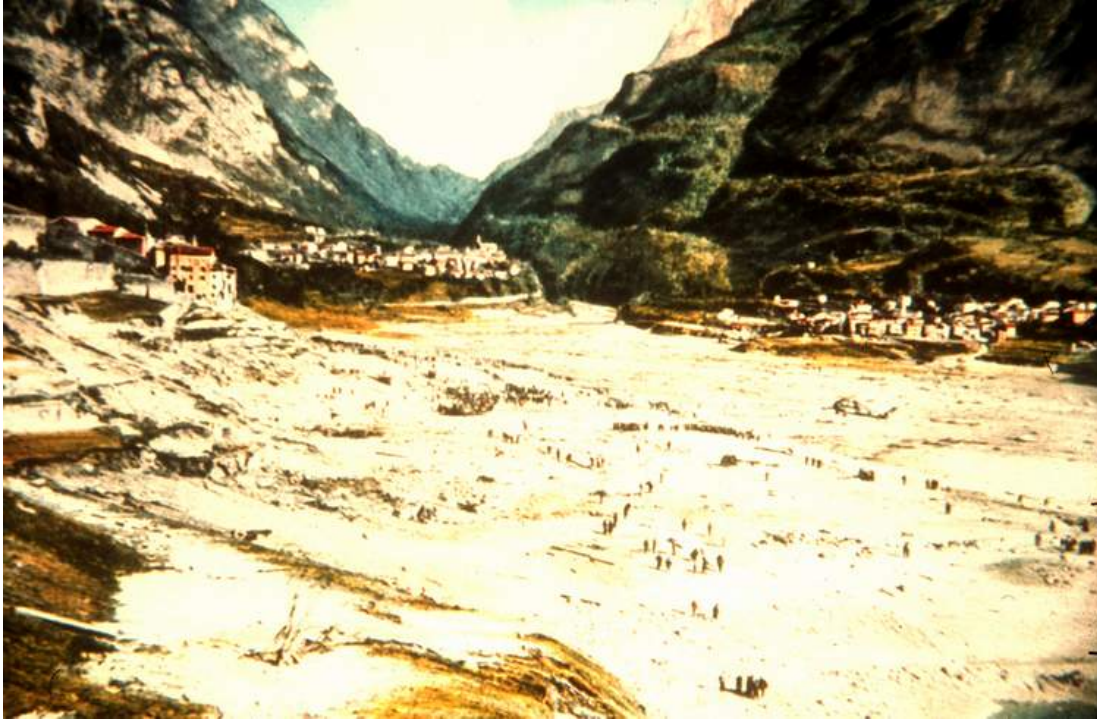
Figure 1.1d: The remains of the town of Longarone after the flood caused by the overtopping of the Vajont dam as a result of the Mount Toc failure. More than 2000 persons were killed in this flood.
