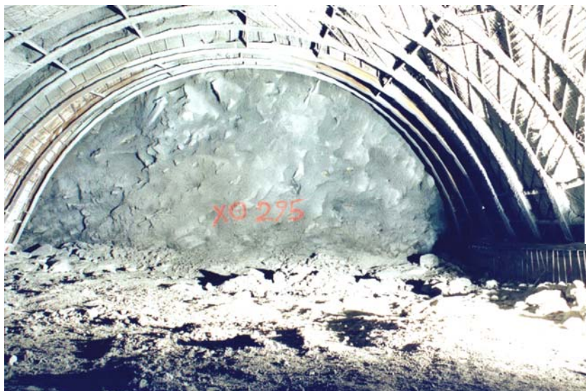
Figure 11.14: Top heading supported by cables and rockbolts and light steel sets.
