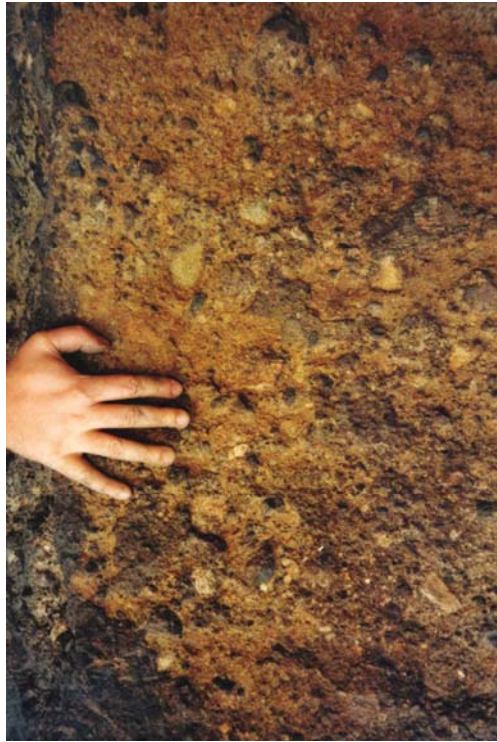
Figure 11.18: Braden Breccia at El Teniente Mine in Chile. This rock is a cemented breccia with practically no joints. It was dealt with in a manner similar to weak concrete and tests were carried out on 100 mm diameter specimens illustrated in Figure 11.19.
