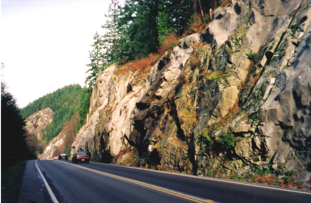
Figure 9.10: The Argillite Cut on Highway 99 in British Columbia, Canada.
