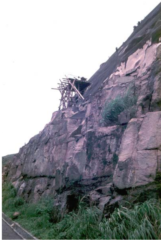
Figure 7.10: Drilling horizontal drain holes into the face of one of the benches of the Sau Mau Ping slope.
