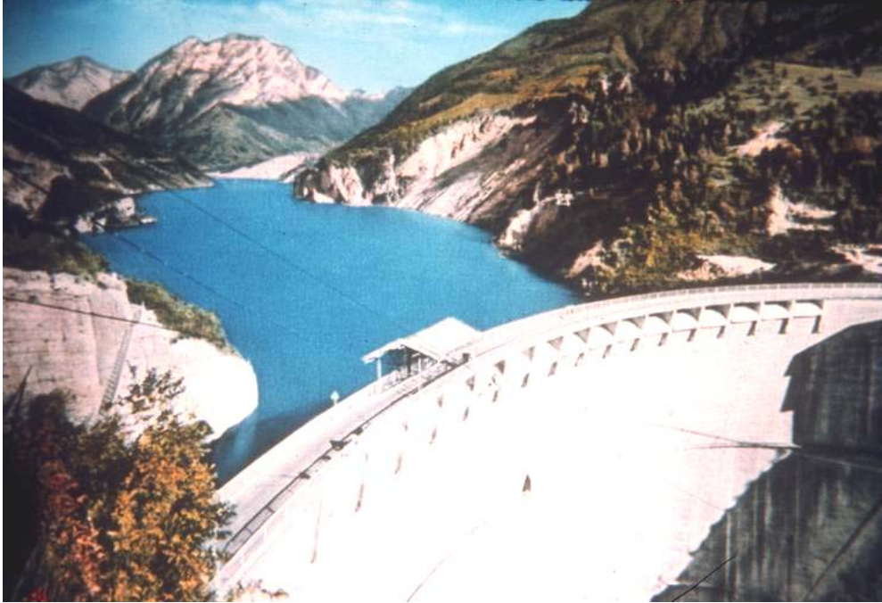
Figure 1.1a: The Vajont dam during impounding of the reservoir. In the middle distance, in the centre of the picture, is Mount Toc with the unstable slope visible as a white scar on the mountain side above the waterline.
