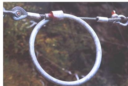
Figure 9.5: Details of a rockfall net system manufactured by Geobruigg of Switzerland.
