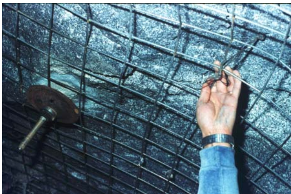
Figure 15.8: Welded wire mesh, firmly attached to the rock surface, provides excellent reinforcement for shotcrete.
