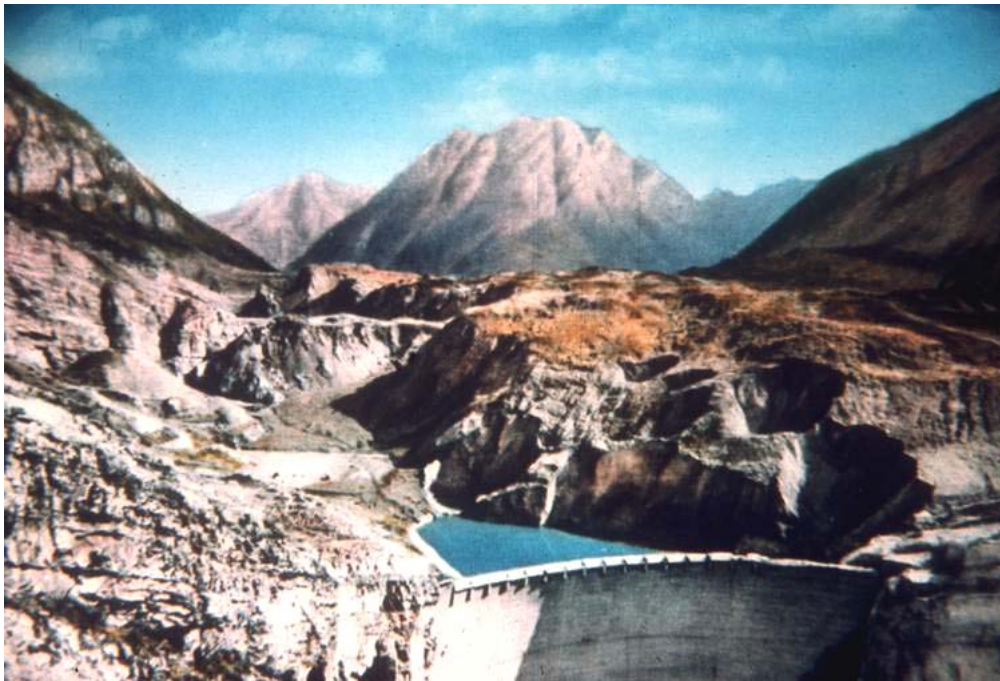
Figure 1.1b: During the filling of the Vajont reservoir the toe of the slope on Mount Toc was submerged and this precipitated a slide. The mound of debris from the slide is visible in the central part of the photograph. The very rapid descent of the slide material displaced the water in the reservoir causing a 100 m high wave to overtop the dam wall. The dam itself, visible in the foreground, was largely undamaged.
