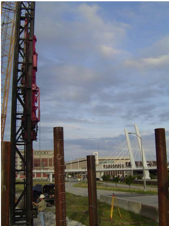
Figure 14. Delmag D46-32 at Static Load Test Site E
