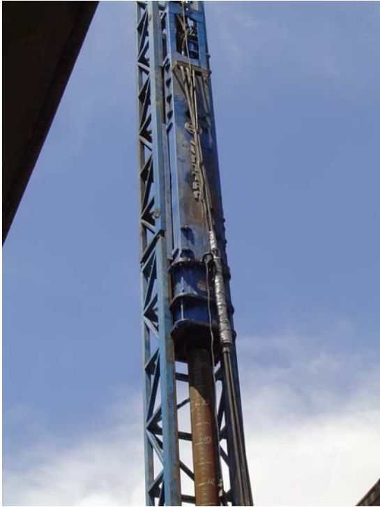
Figure 15. Junttan HHK 10A driving a pile on a non static load test site
