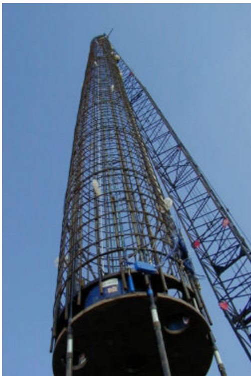
Figure 5.4 Load cell in reinforcement
