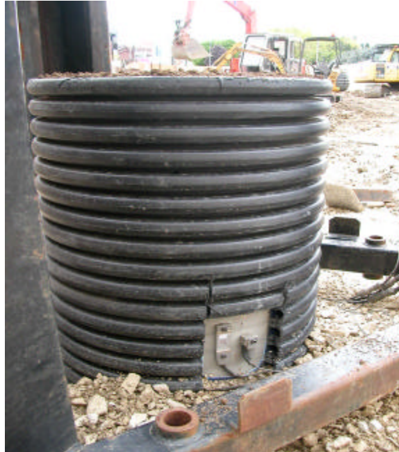
Figure 5.10 Bored cast in place/CFA pile head preparation with window cut in liner to allow strain gauge and accelerometer to be attached to the pile
