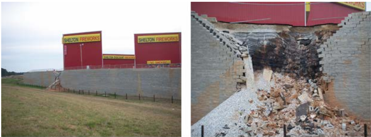
Figure 1-3. Geosynthetic reinforced wall: limit state shallow failure [I-85 near Exit 70, Cusseta, Alabama; photo taken February 2007]
