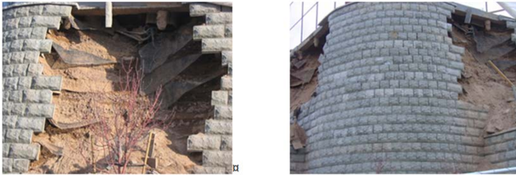
Figure 1-1. Result of missing reinforcement: close-up (left) and general view (right) [January 2008, Salt Lake City, Utah]
