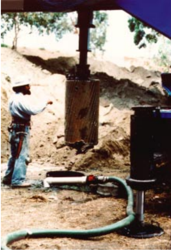
Figure 6-4: Drilling Bucket
