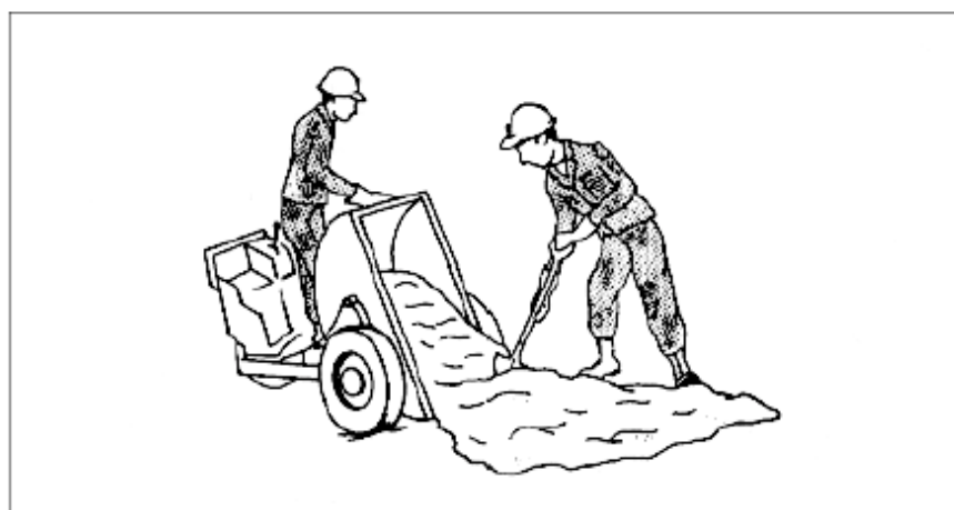
Figure 5-8. Handling concrete by power buggy
