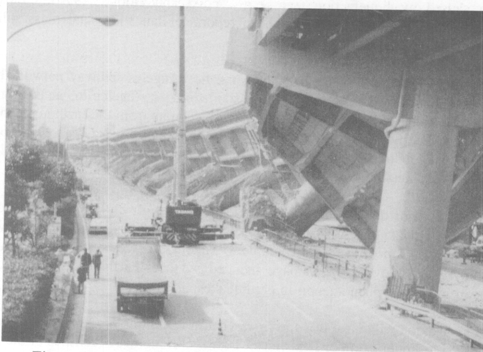
Figure 5. Collapse of Hanshin expressway during the 1995 Kobe (Hyogo-Ken Nabe, Japan) earthquake.
