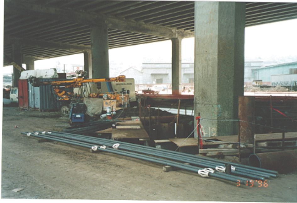
Photograph 8 - 2. Storage of Reinforcing Steel
