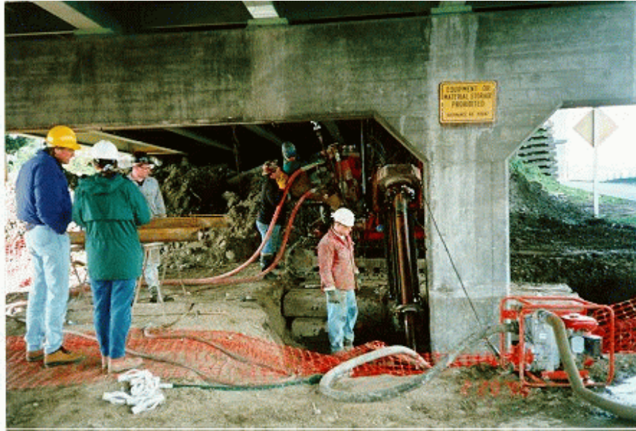
Photograph 3 - 5. Low Headroom Micropile Installation
