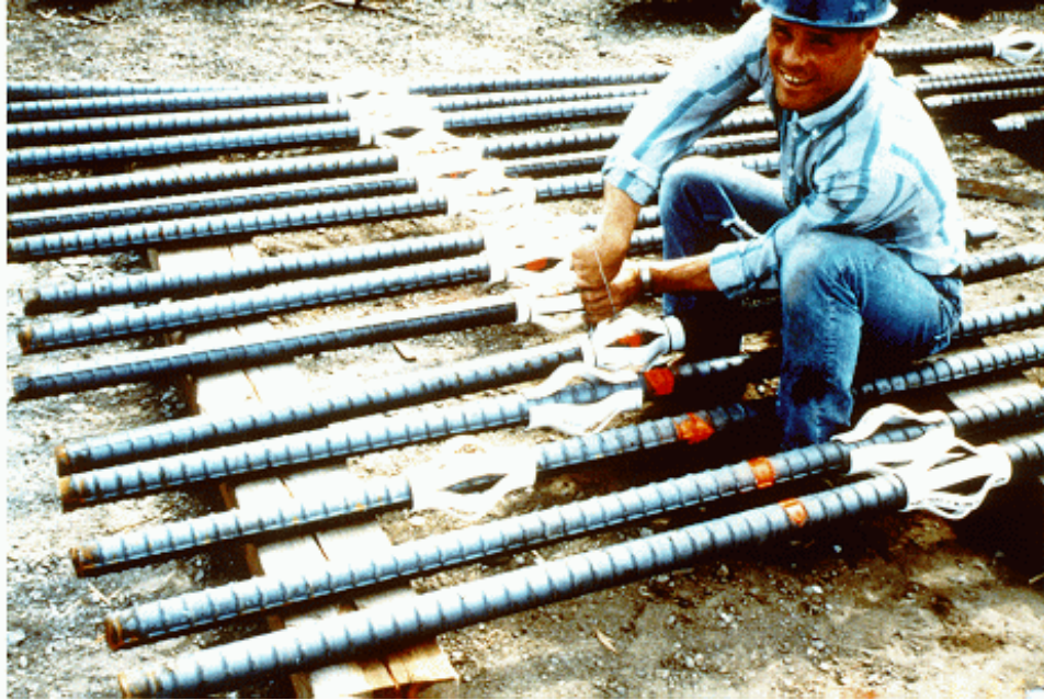
Photograph 8 - 5. Reinforcement Centralizers
