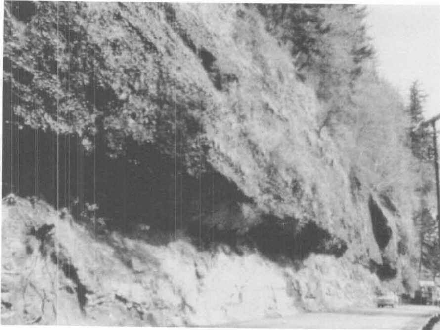
Figure 3.5 110-foot high slope.
