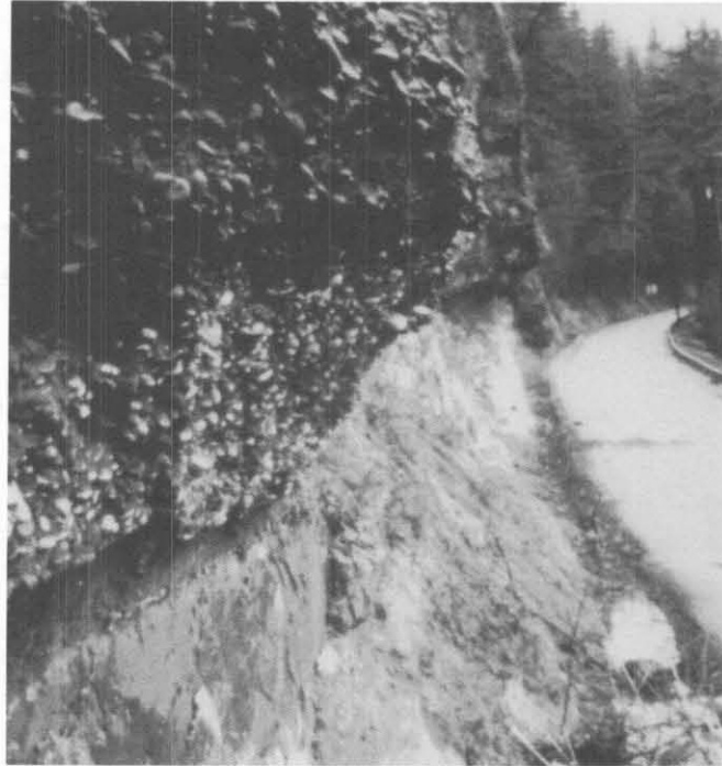
Figure 5.11 The measured sight distance is 330 feet.
