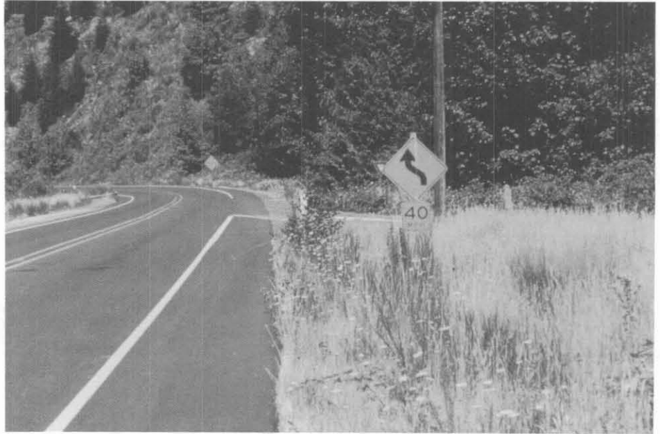
Figure 5.8 Roadway curves with reduced posted speed limits are common in rugged terrain. Remember to record this information.
