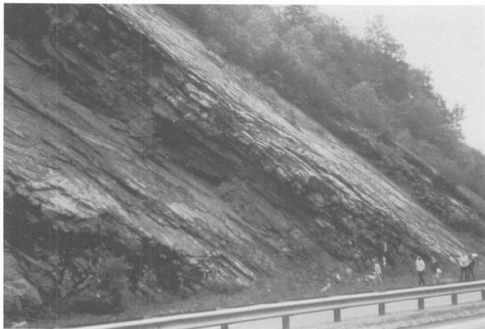
Figure 5.17 Continuous joints with adverse orientation.
