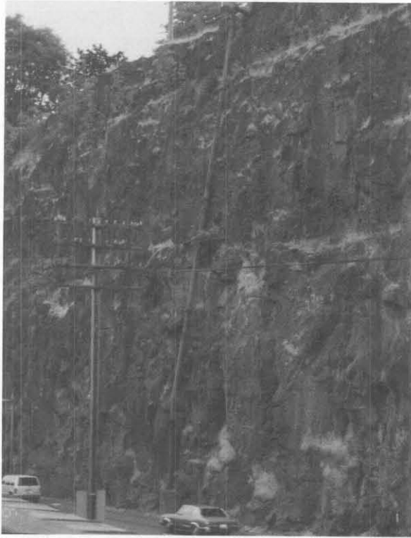
Figure 5.2 When the slope is nearly vertical and there is access to the top, the height can be measured with a tape.
