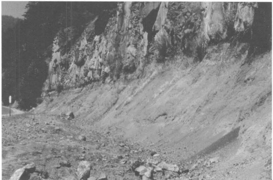
Figure 3.2 "B" rated slope.
