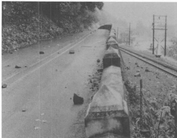
Figure 5.10 Vertical curves can also restrict sight distance.
