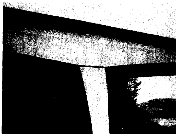
Figure 8. Closeup of bridge shown in figure 10 showing no signs of distress in spite of differential settlement of abutment.
