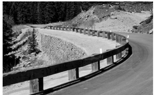
Figure 2-23. Guanella Pass architectural concrete faced wall.
