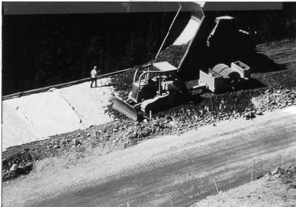
Figure 11-7. Placement of reinforced fill.
