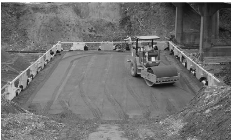
Figure 2-10. Compaction of the reinforced wall fill.
