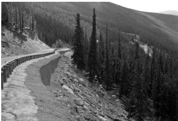
Figure 2-22. Guanella Pass wire-faced wall.
