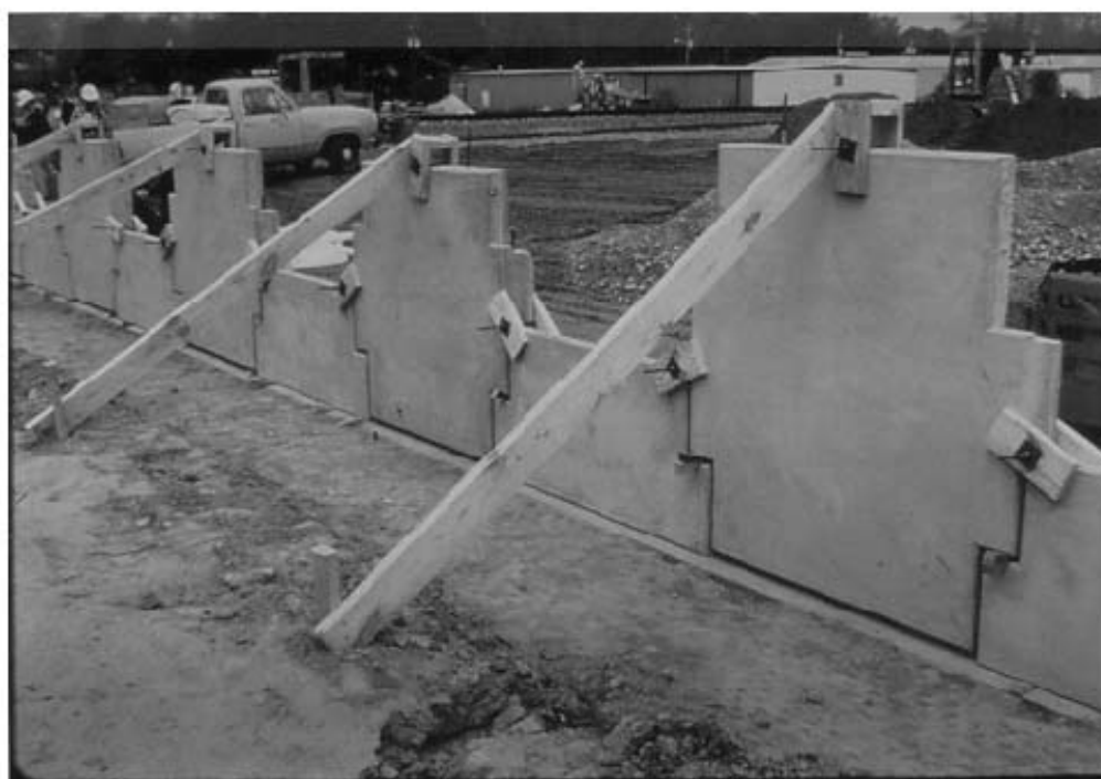
Figure 11-6. Setting first row of precast facing elements.
