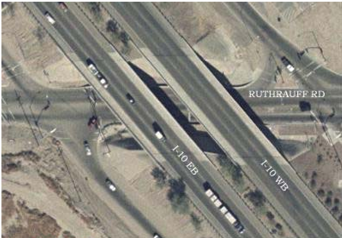
Figure 1-1. Aerial view of a pair of 3-span Interstate 10 (I-10) bridges over a local roadway in Tucson, Arizona.
