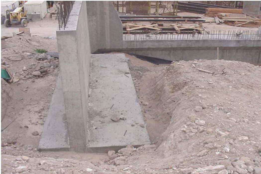
Figure 8-5. Abutment/wingwall footing, I-10, Arizona.
