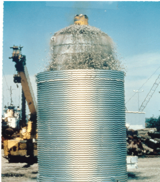
Figure 9-77. Photograph of Statnamic ® test arrangement showing masses being accelerated inside gravel-filled sheath.
