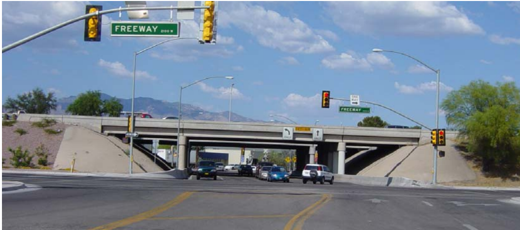
Figure 1-2. Example of 3-span roadway bridges over another roadway.
