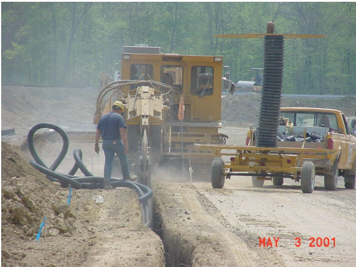
Figure 8-4. Underdrain installation ( photo courtesy of Ohio DOT ).
