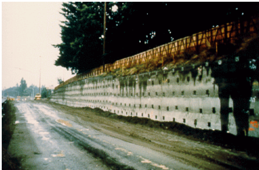
Figure A-2. Black Lake Interchange, WSDOT Olympia, WA - Soil Nail Wall Construction
