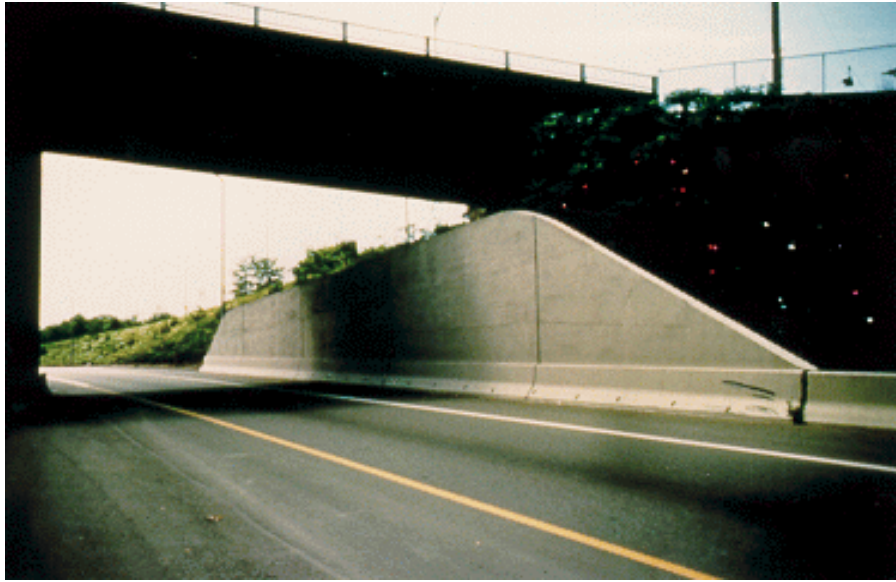
Figure A-5. I-5, WSDOT Tacoma, WA - Soil Nail Wall in Tacoma (Bridge End Slope Removal)
