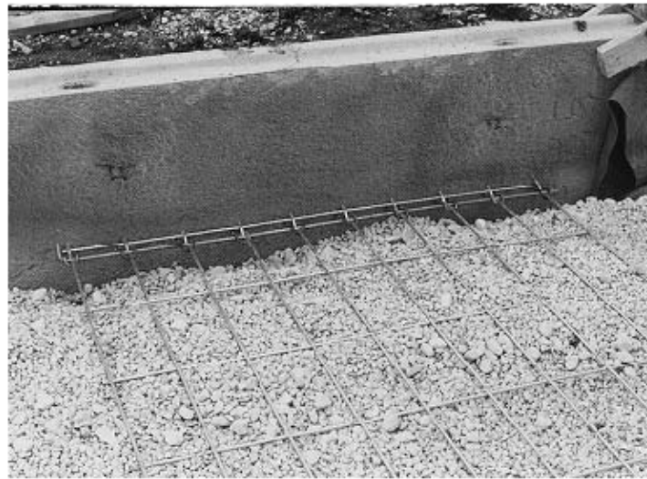
Figure 3. Photo. MSE inextensible reinforcement—wire mats. (3)
