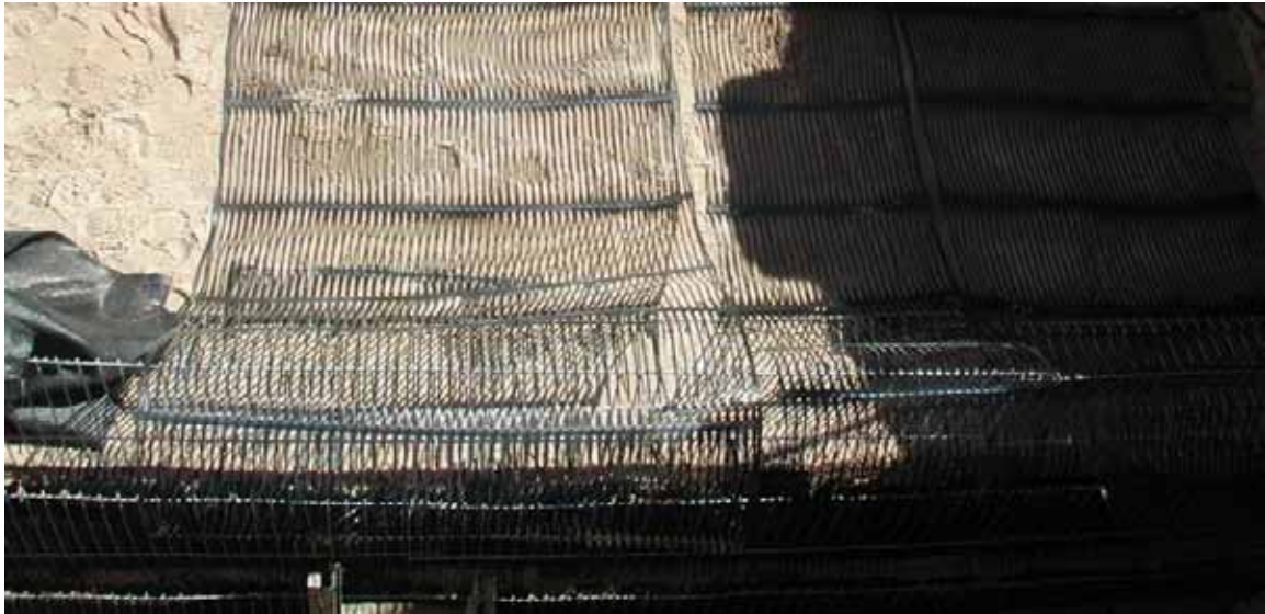
Figure 4. Photo. MSE extensible reinforcement (geogrid).
