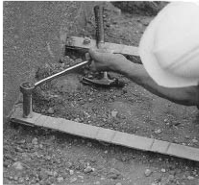
Figure 2. Photo. MSE inextensible reinforcement—steel strips. (3)
