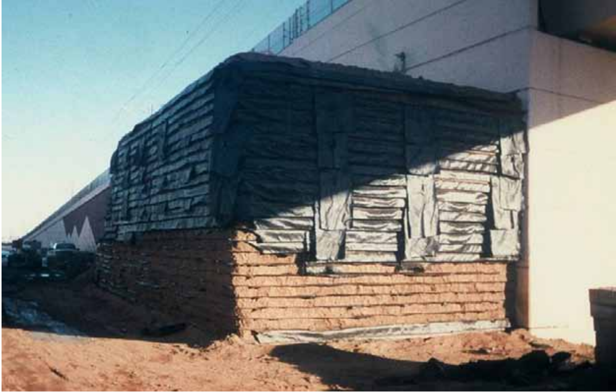
Figure 8. Photo. Internally supported GRS structure.
