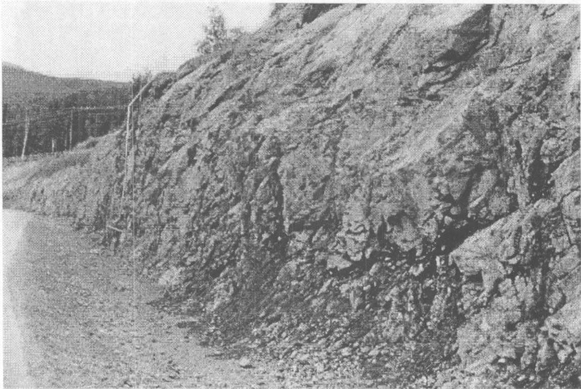
Figure 11.4A Blast Without Presplit (Siltstone, Alaska)
