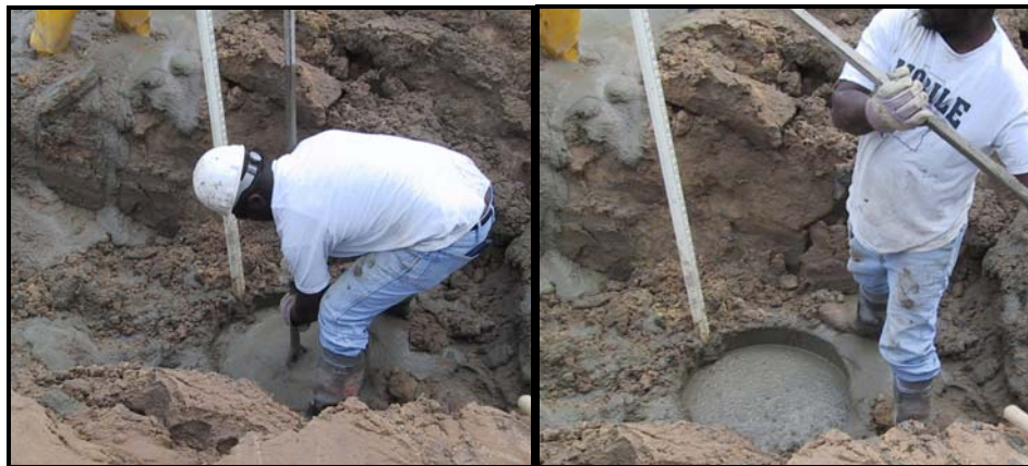
(c) and (d) Contaminated Grout Removal
