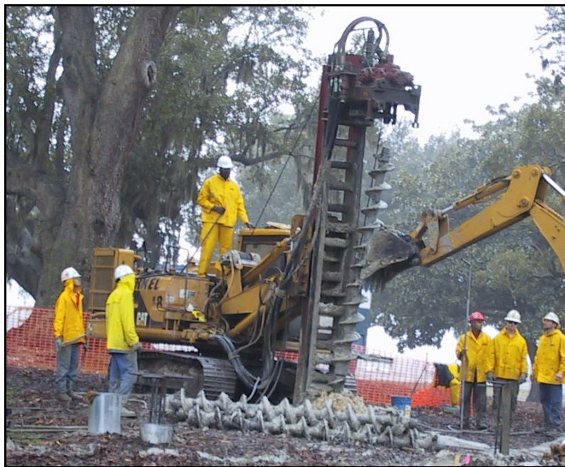
Figure 4.4: Low Headroom Rig with Segmental Augers
