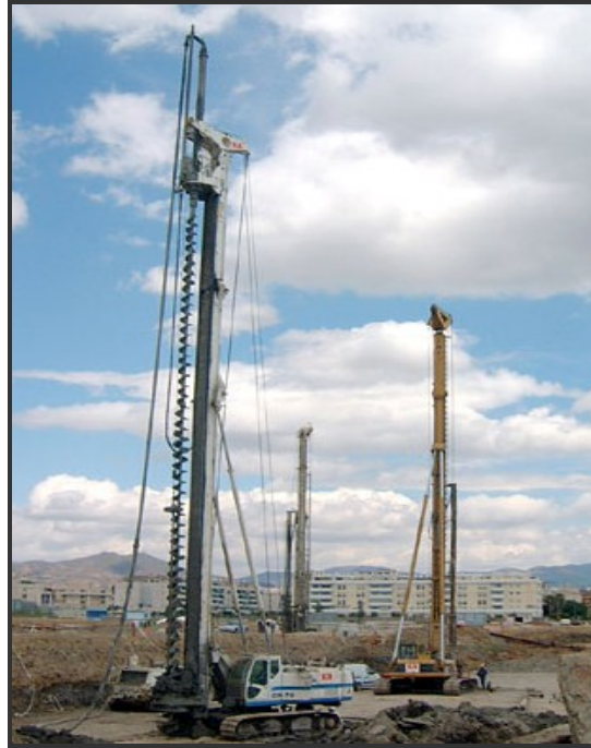
Figure 4.6: Soilmec Hydraulic CFA Rig with Kelly-Bar Extension
