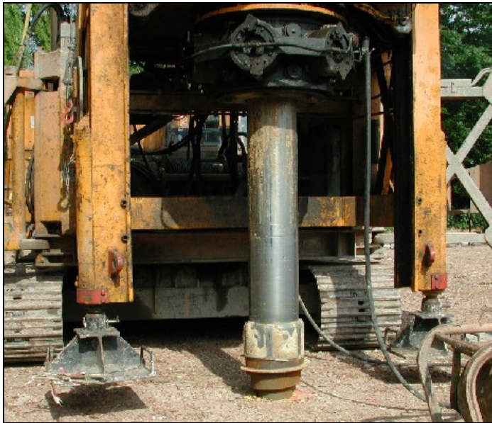
Figure 4.13: Fundex Screw Pile
