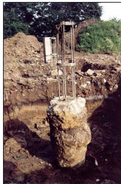
Figure 4.13: Fundex Screw Pile
