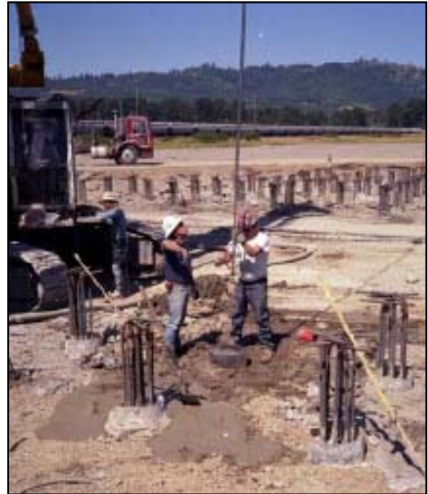
Figure 2.11: Placement of a Single Full-Length Bar
