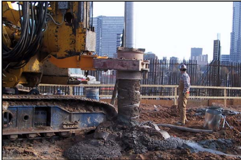
(a) Full Displacement Pile
