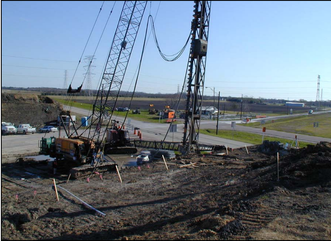
Figure 3.11: CFA Piles at the Krenek Road Bridge Site
