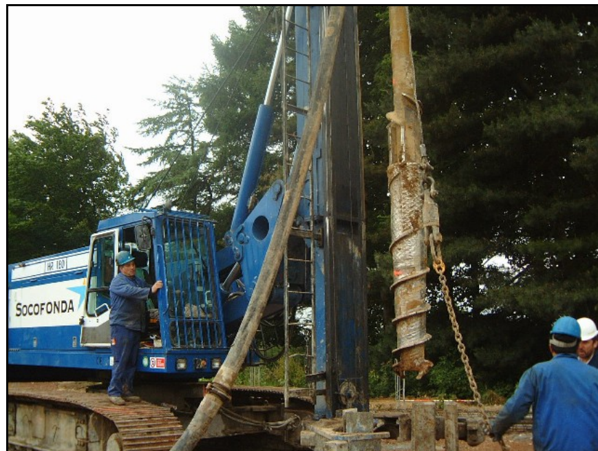
Figure 4.12: Omega Screw Pile
