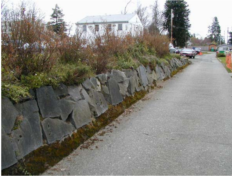
Figure 13. Photograph. Single-tier, 1.2-m (4-ft) rockery near state capital building, Olympia, Washington (Site 3).
