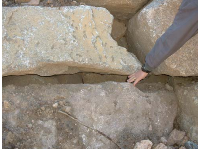
Figure 68. Photograph. Example of an unacceptable rock bearing.
