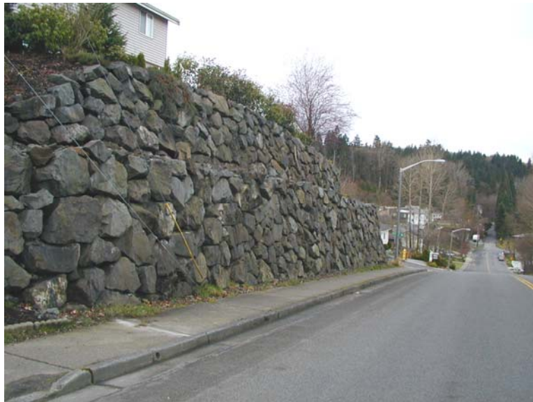
Figure 12. Photograph. Two-tier, 7.3-m (24-ft) rockery, 15th Avenue at 12th Street, Puyallup, Washington (Site 2), with guy wire anchored at base of rockery.
