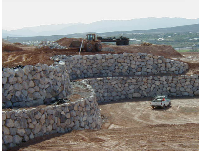
Figure 20. Photograph. “Protecting” rockery used as a facing for a 9.1-m-high (30-ft-high) MSE wall with a 5.5-m (18-ft) maximum tier height in Henderson, Nevada (2001).
