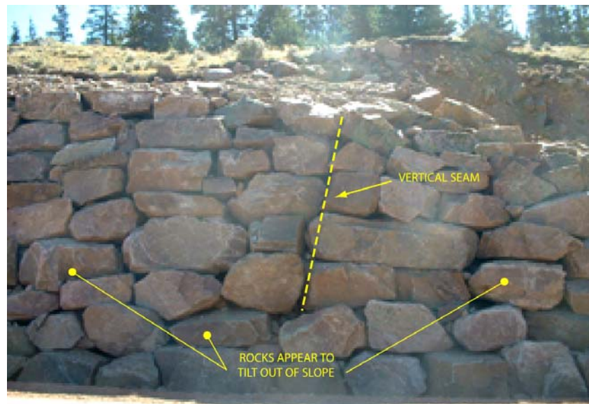
Figure 75. Photograph. Example of improper rockery layout evidences by vertical seams and rocks inclined out of face.
