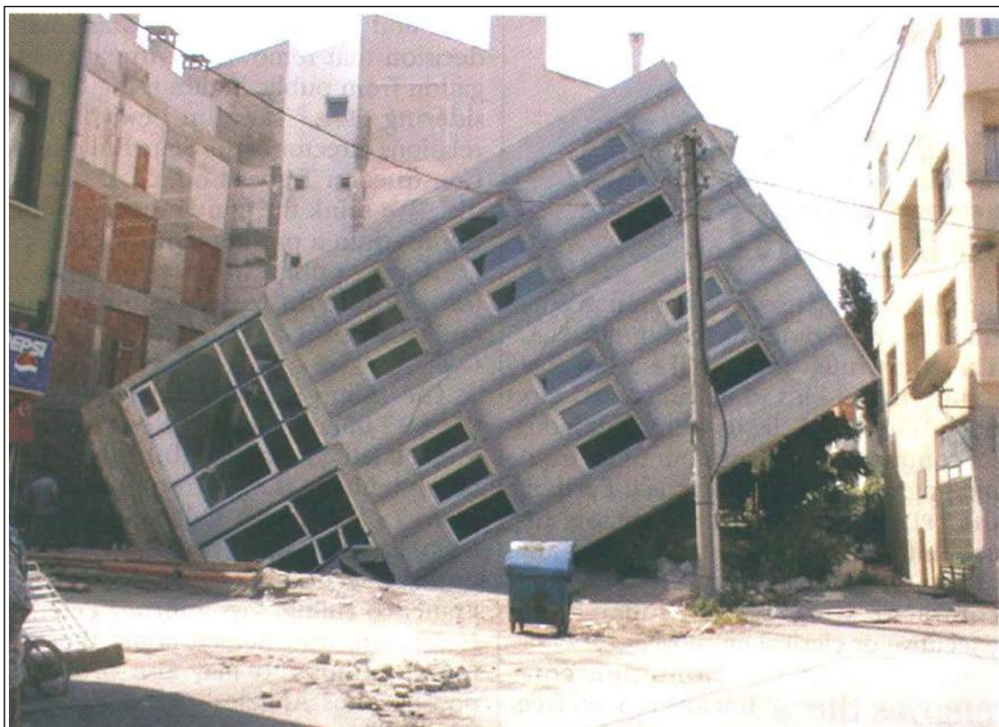
Fig. 2.27 Effect of liquefaction from the 7.4 Magnitude Kocaeli Earthquake of August 17, 1999 in Turkey. Courtesy of Dr. N.J. Gardner, University of Ottawa.
