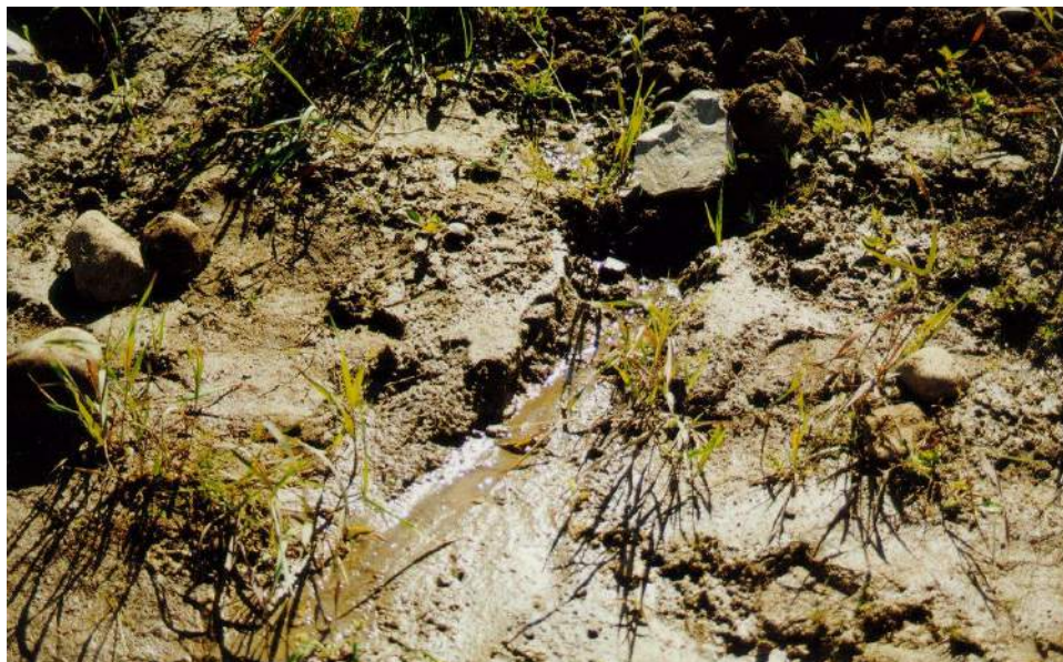
Fig. 4.8 Water discharging from a drain immediately outside the embankment
