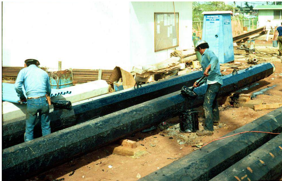
Fig. 7.33 View of applying a bitumen coat to a concrete pile
