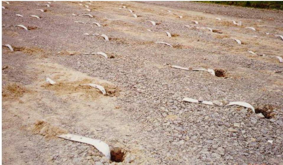
Fig. 4.7 View over a site after completed wick drain installation
